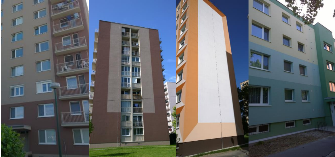
Figure 4.4 Building envelope after thermal insulation implementation (Source: Author)
