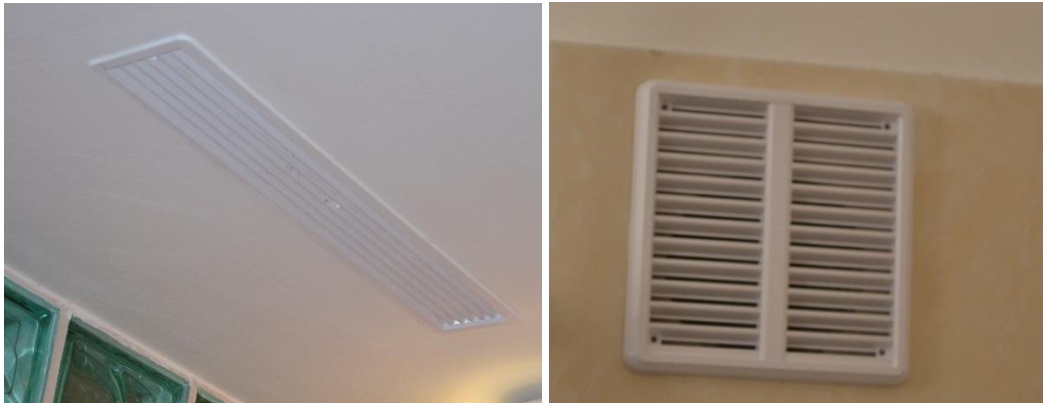
Figure 4.6 Exhaust ventilation in sanitary rooms (Source: Author)
