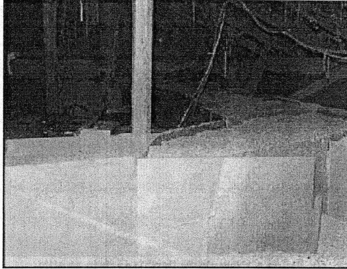
Figure 6. Blown in place duct insulation
