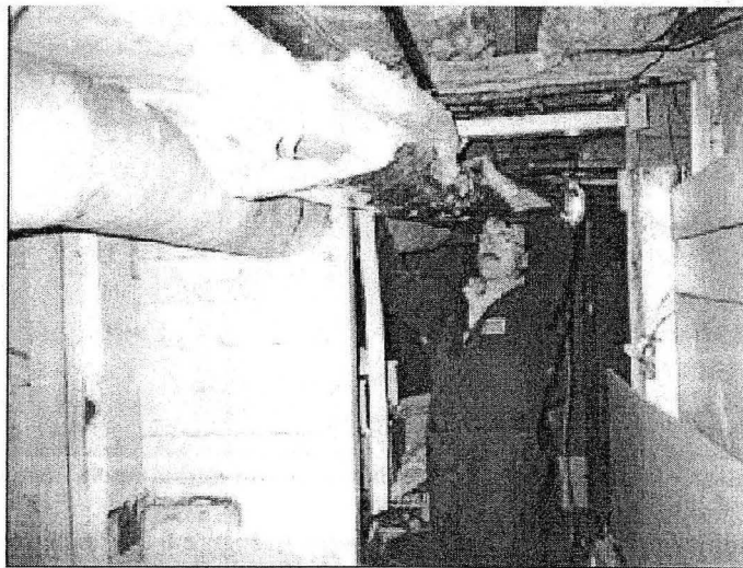
Figure 7. Installing extra duct insulation
