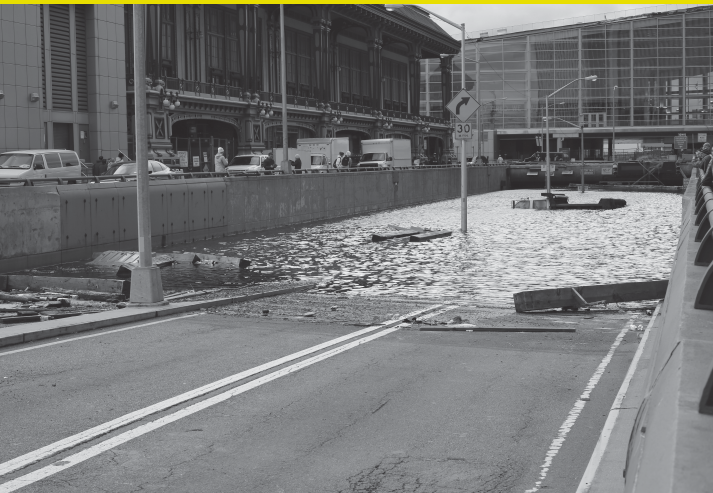
BATTERY PARK, MANHATTAN Flooded Tunnel after Hurricane Sandy (PHOTO: TIMOTHY KRAUSE)
