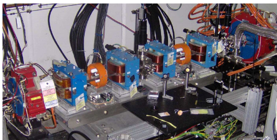
Figure 4: Image of C2 after installation.
