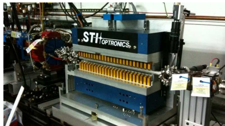
Figure 5: Image of U2 after installation.
