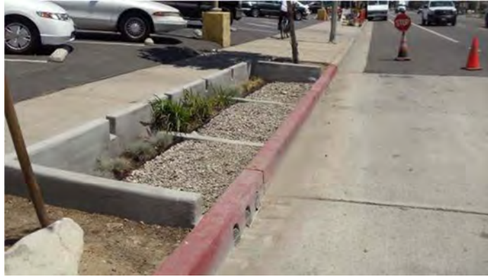
Photograph of a grassy swale under construction.
