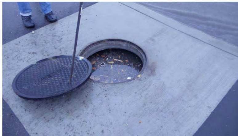
Photo of a catch basin during a sampling event before entering a percolation well.
