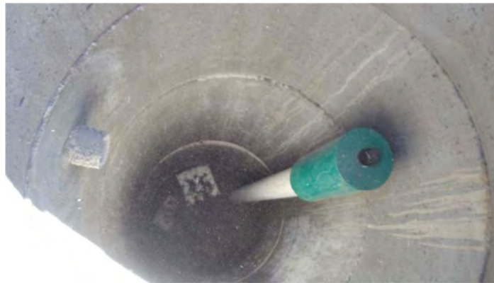
Photograph shows the secondary chamber of a finished dry well.
