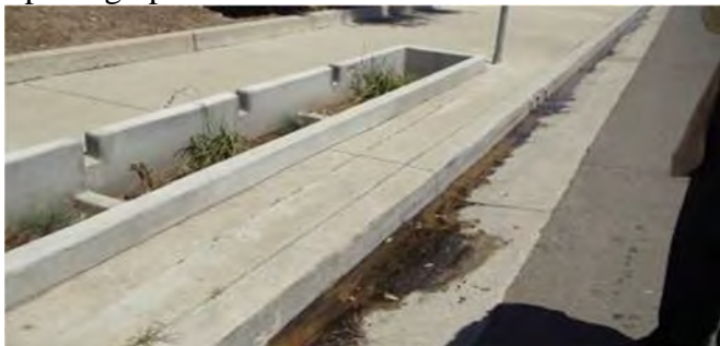
Photograph shows formed concrete for a grassy swale.
