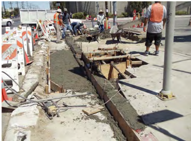
Pouring the concrete for the dry wells and catch basin site.
