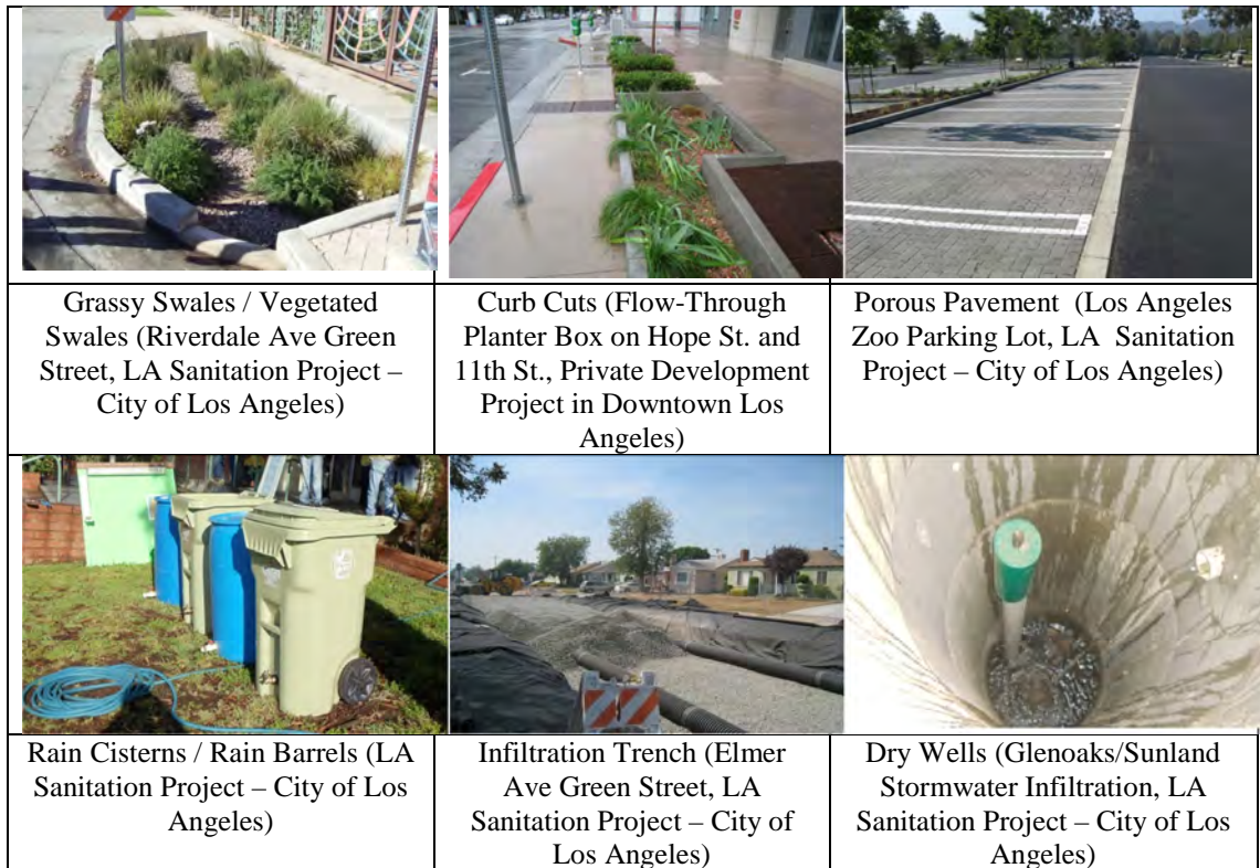
Figure 2. Several Stormwater Control Measures (SCMs) that capture rain and retain runoff) in City of Los Angeles.
