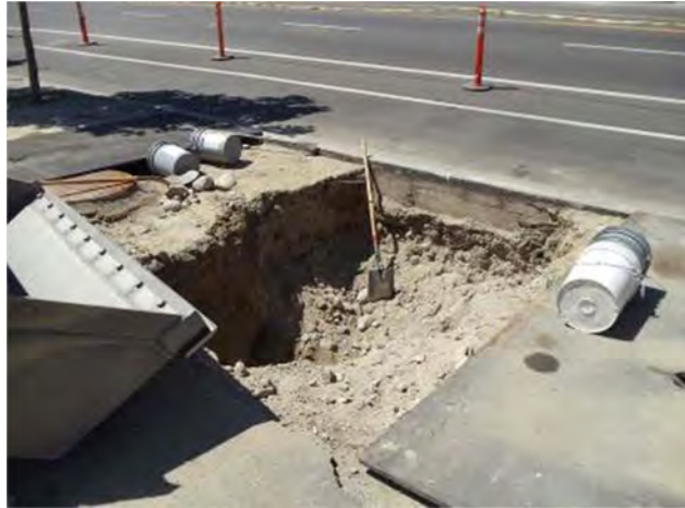
This photograph shows excavation in a grassy swale.
