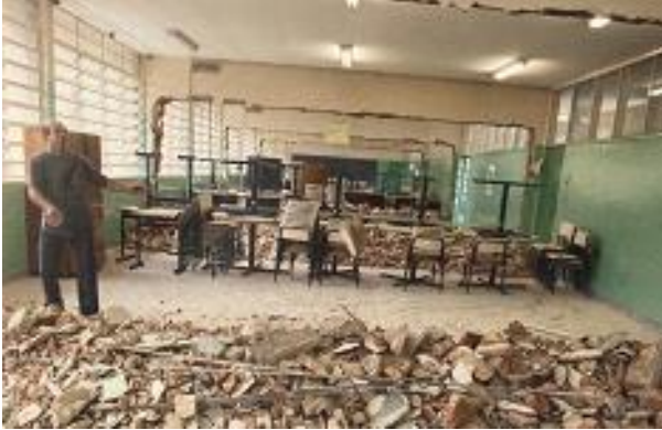
Historical picture depicting the former principal Braz Nogueira and the demolition of internal classroom walls. This photograph was captured from a mural on the history of the Bairro Educador (Educational Neighborhood) at the CEU Heliópolis complex.
