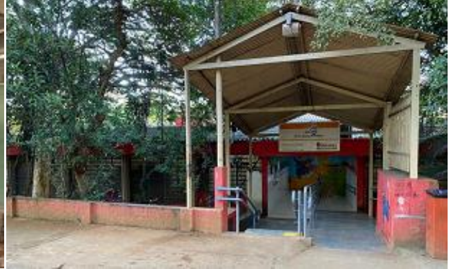
EMEF Campos Salles school front entrance. The image highlights the removal of the external walls.
