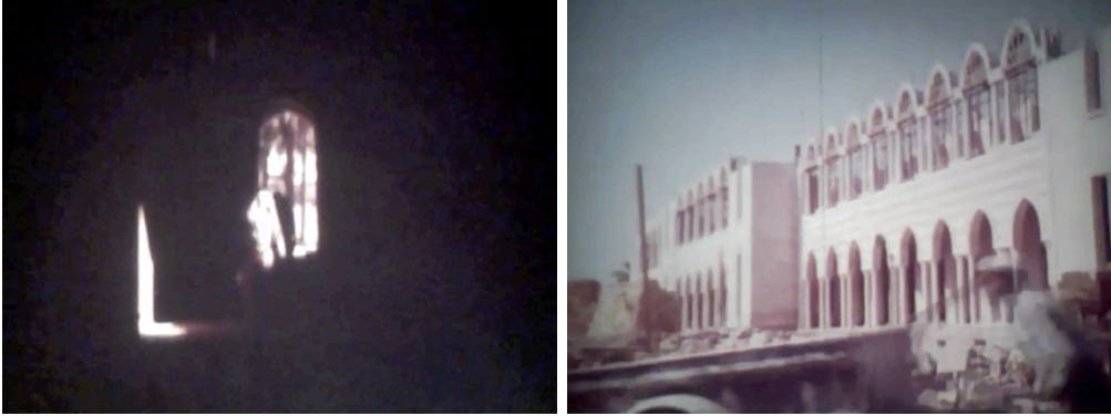
Figure 5.18 Stills from transition from old Baghdad (dark) to new construction of new Parliament building (light) in A More Beautiful Capital
