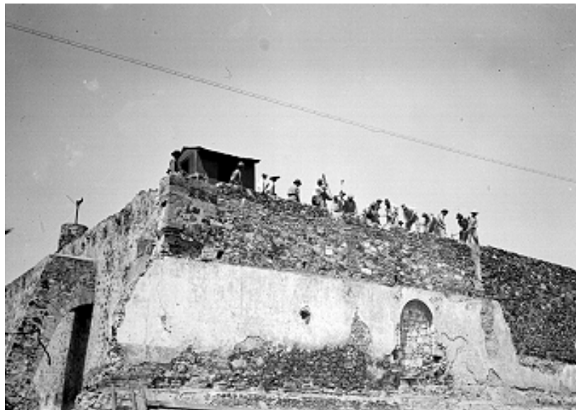
FIGURE 26. “Workers demolishing the Cárcel de Belem.” 420 Courtesy of the INAH.
