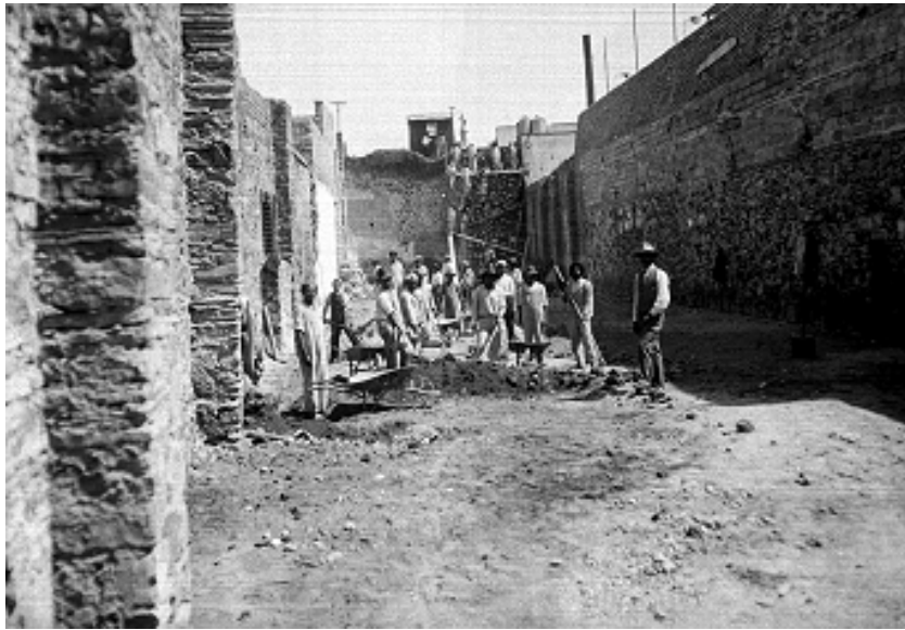
FIGURE 25. “Workers during the demolition of the Cárcel de Belem.” 419 Courtesy of the INAH.
