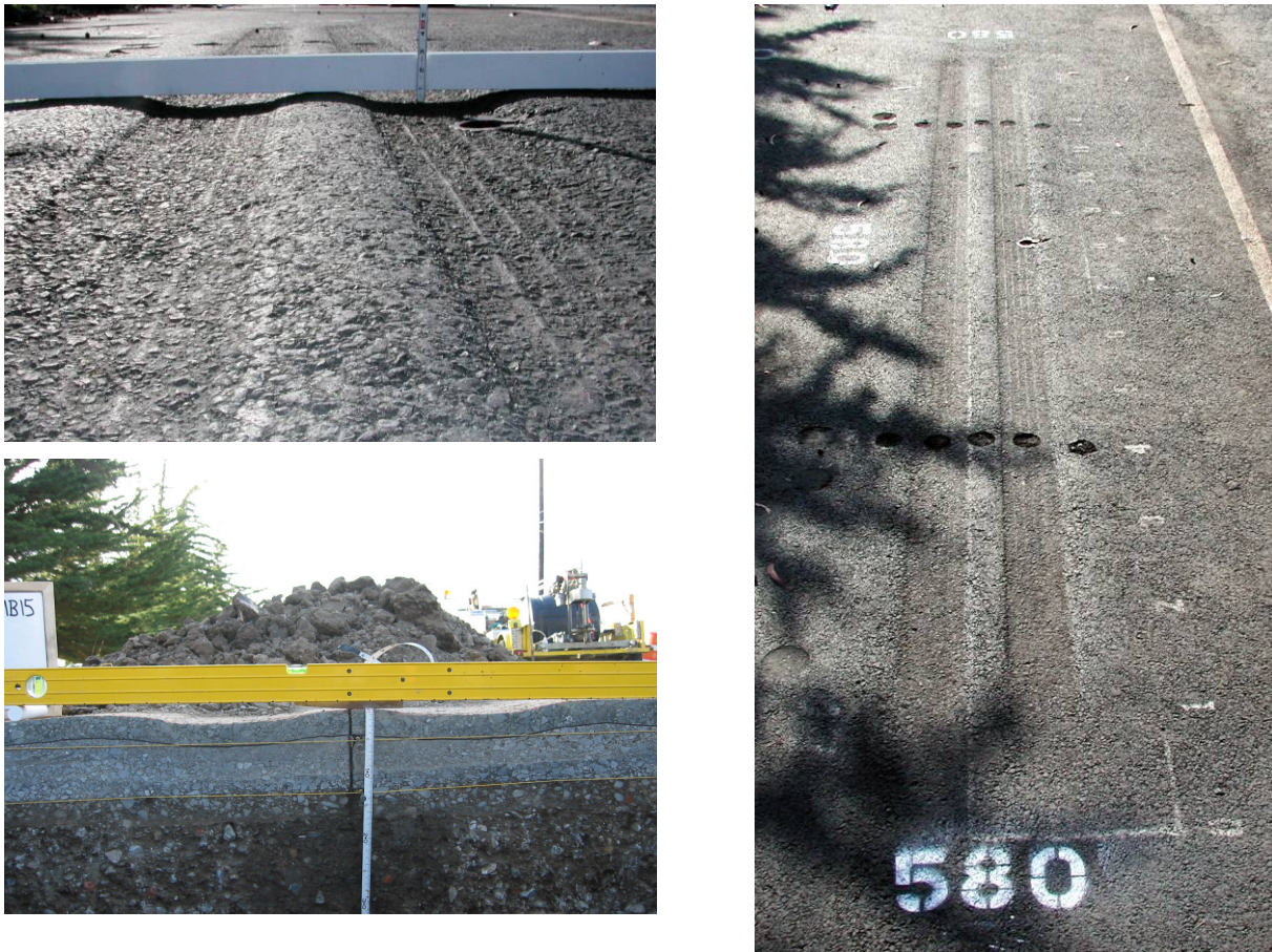
Figure 3.13: 580RF: Section photographs at the end of the test.
