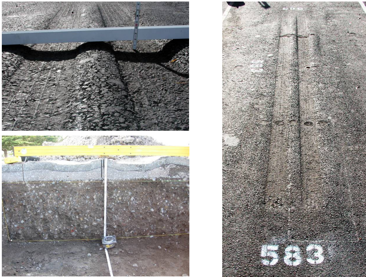
Figure 3.46: 583RF: Section photographs at the end of the test.
