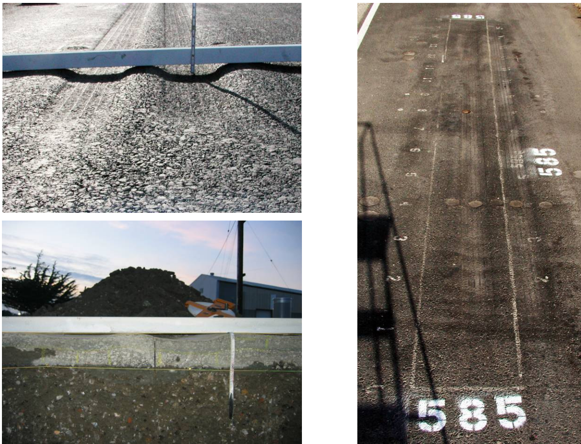
Figure 3.68: 585RF: Section photographs at the end of the test.
