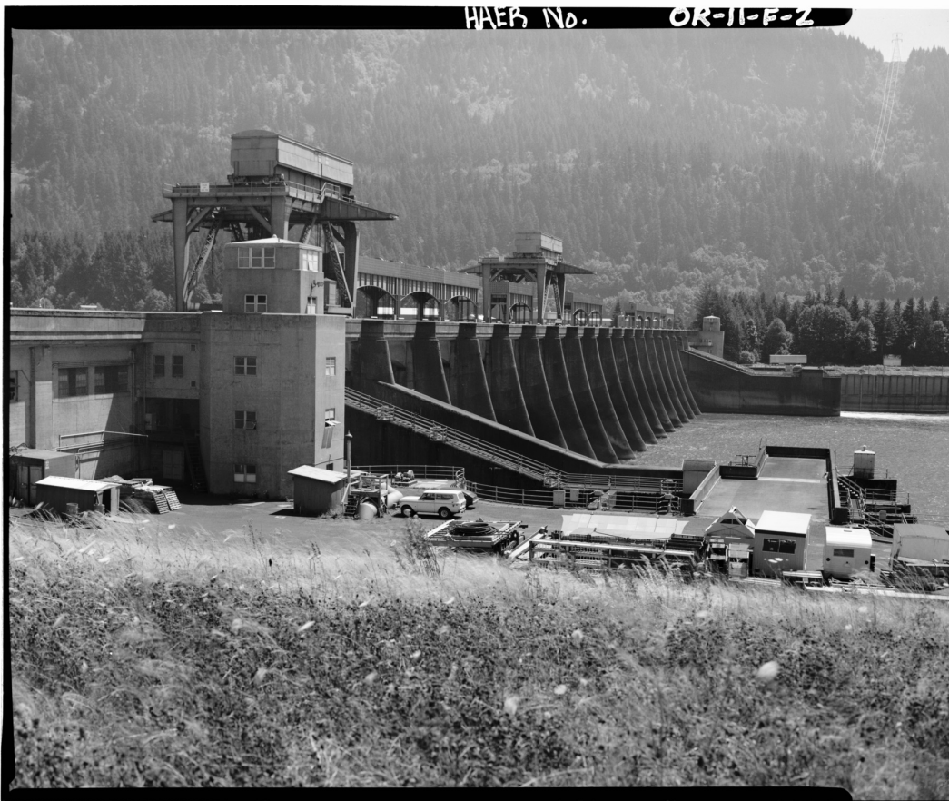
Fig. 7: Downstream Face of the Spillway (from Cascades Island, looking south). National Parks Service.
