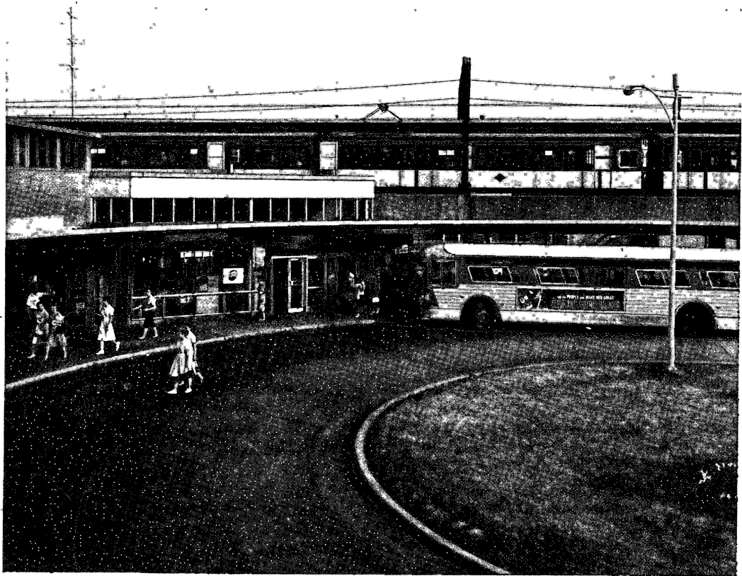
Fig. 10.2 — Windermere Terminus, Cleveland Rapid Transit, showing off-street loop and shelter for feeder buses.
