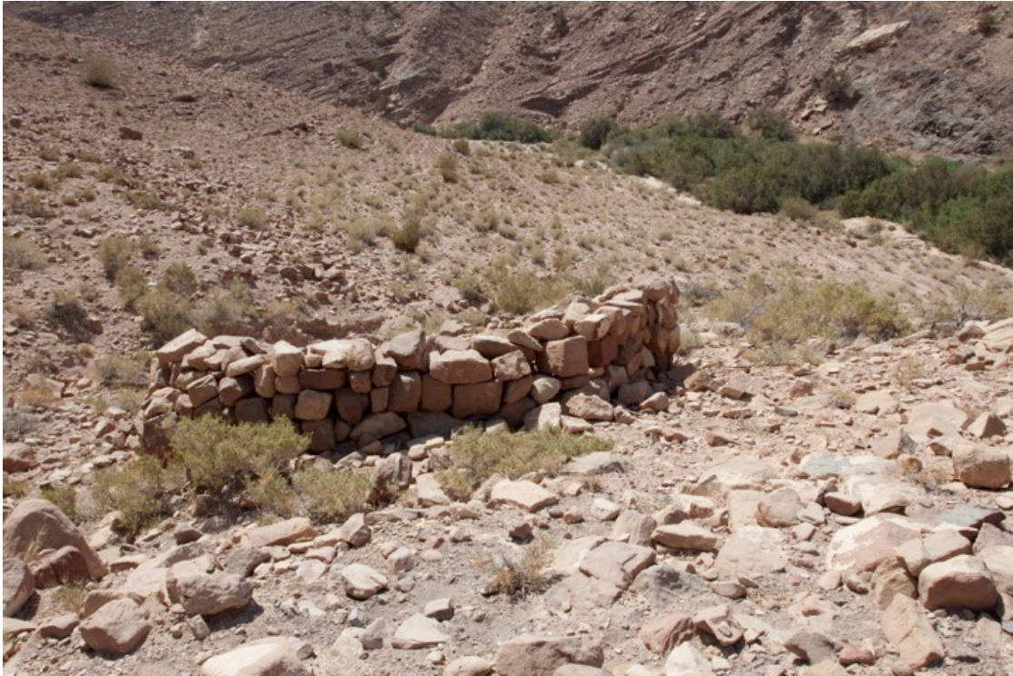
Figure 2.12: Site 114 (Khirbat Feidh) a Roman period site that is very poorly preserved. Many terrace walls and other derelict structures were recorded here, suggesting its use for agriculture. New structures have also been built by modern inhabitants of the valley for shelter and for animal penning.
