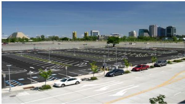
Figure: 4.3 Location for Asphalt based Analysis (A hypothetical location similar to Sacramento bridge area parking lot was considered for the simulation area in EnviMet)
