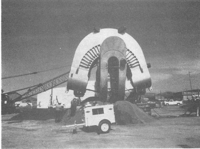
Photo. 17. (CBB 831-892). Coil box assembly of superconducting Yin-Yang magnet for Mirror Fusion Test Facility (MFTF) LLNL photo.
