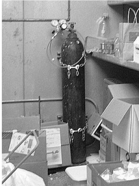
Figure B.5: Smaller tank restraint
