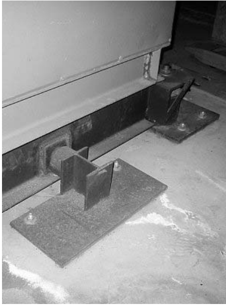
Figure A.5: Seismic bracing
