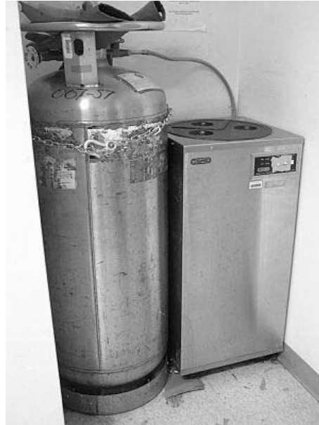
Figure B.6: Larger tank restraint
