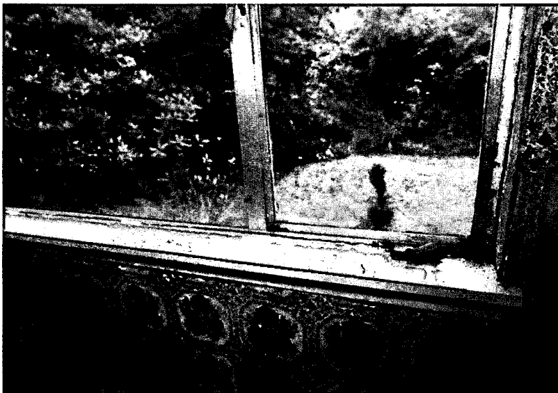
Single-glazed windows characteristically suffer from water condensation problems and the formation of frost on the inside surface of the glass in winter.
