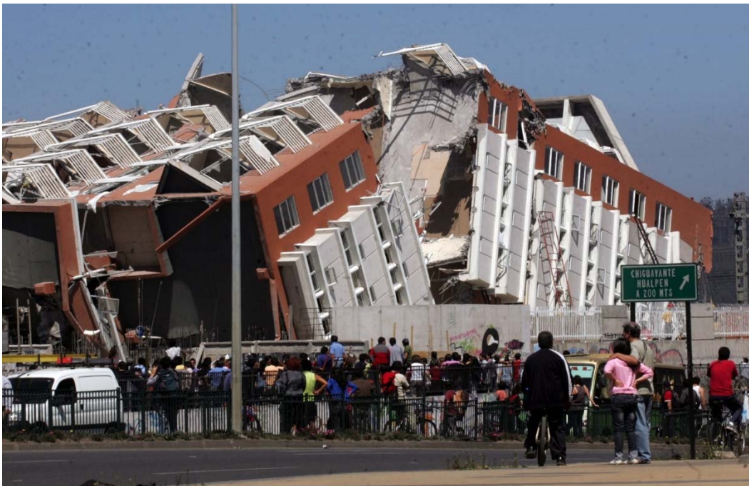
Figure 6.66 Collapse of Alto Rio building following 2010 Maule earthquake, after IDIEM (2010).
