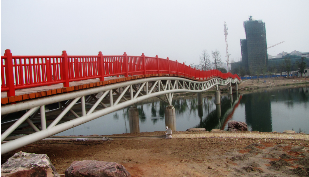
Fig. 2. Overview of the Fenghe Bridge.
