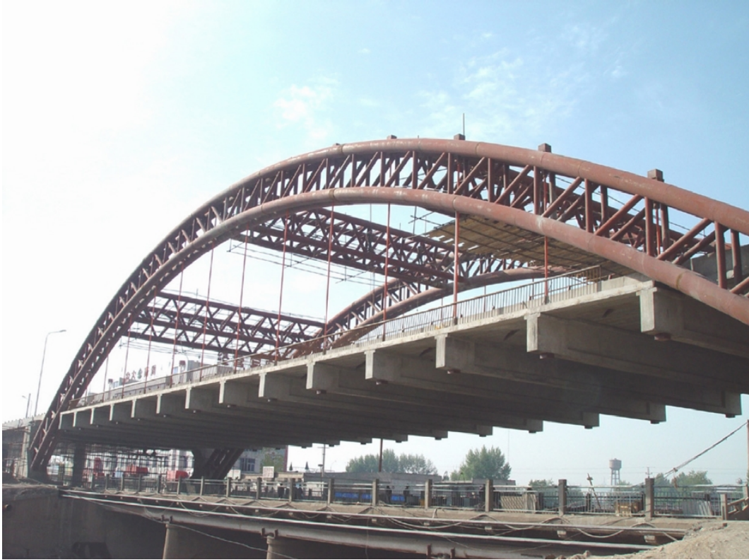
Fig. 7. General view of the Beichuan River Bridge.
