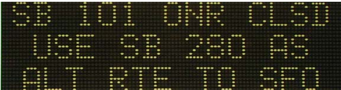
Figure 11A: A compacted permanent CMS sign.
