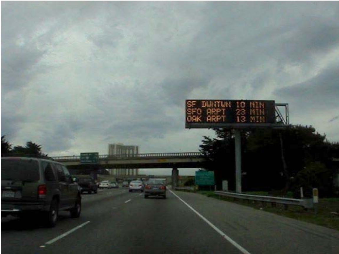
Figure 2: The permanent CMS used for the test as it looks from the rightmost lane (this picture was not taken at test time).
