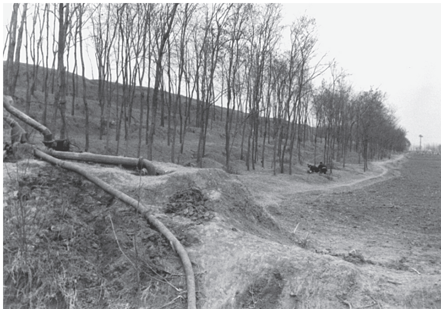
Fig. 28. The Walls of Qufu (Shandong). First constructed during the Late Western Zhou or Springs and Autumns period and frequently repaired at least through the Hān period. The photograph shows a section of the south wall that was not reused as part of the enclosure of the Ming dynasty Qufu county seat (see Map 9).
