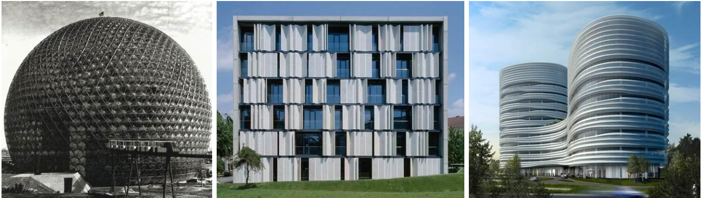
Figure 3: 1a Buckminster Fuller, United States Pavilion , (1967), photo by Rudy Godinez, 1b Bio-tech building at TU Graz , Fertigstellung 2004 . Photo by Paul Ott, 1c CJ Research Center's Kinetic Folding Facade 2012 / Yazdani Studio , photo by Andrew Michler
