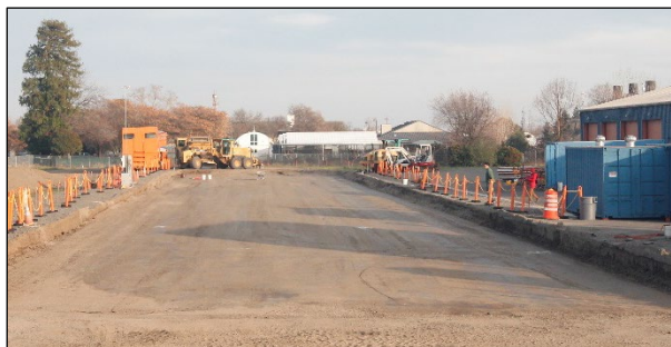
Figure 4.5: Subgrade: Completed preparation.
