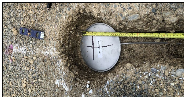
Figure 5.4: Pressure cell installation.
