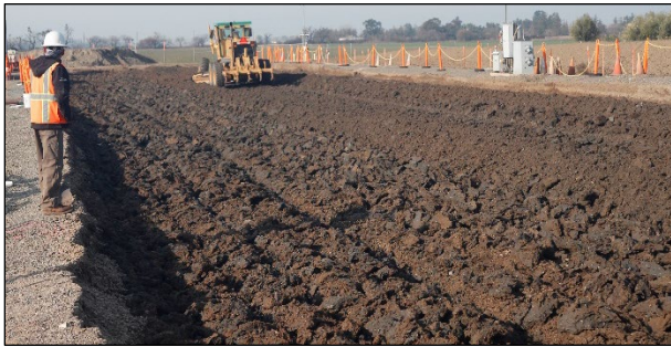
Figure 4.1: Subgrade: Ripping with a grader.
