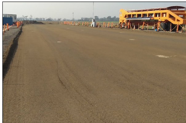
Figure 4.15: Base: Completed preparation.
