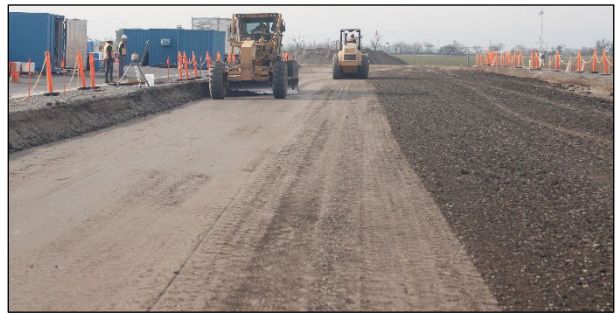
Figure 4.4: Subgrade: Final shaping and compaction.
