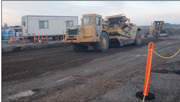
Figure 4.6: Subbase: Importing and spreading material with a scraper.
