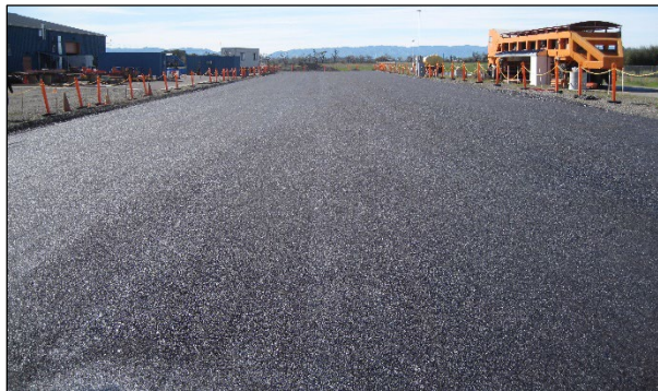
Figure 4.18: Base: Completed prime coat application.
