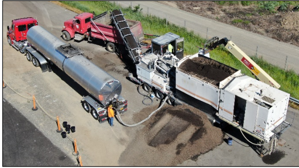
Figure 4.23: CCPR: Belt-feed of processed material to truck.
