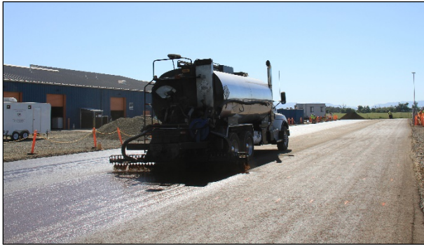
Figure 4.29: CCPR: Curing seal application.
