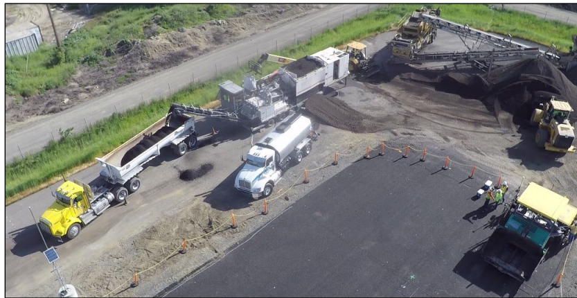
Figure 4.22: CCPR: Central plant setup.
