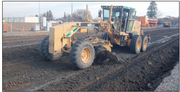
Figure 4.2: Subgrade: Mixing and shaping.
