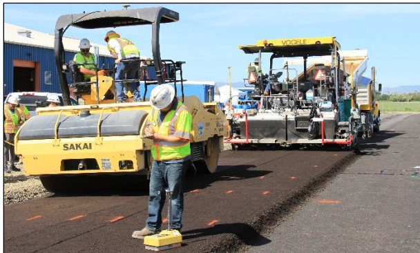
Figure 4.25: CCPR: Paving and breakdown compaction.
