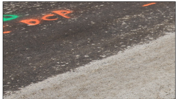
Figure 4.28: CCPR: Crack-free surface after final compaction.
