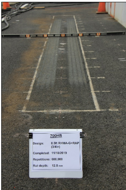
Figure 11.16: 700HB: Test section view from Station 0.
