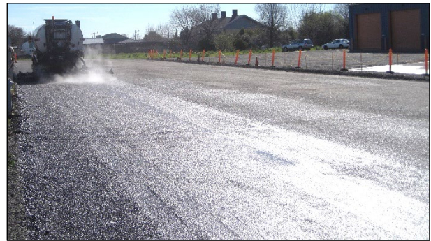
Figure 4.17: Base: Prime coat application.
