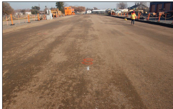
Figure 4.10: Subbase: Completed preparation.
