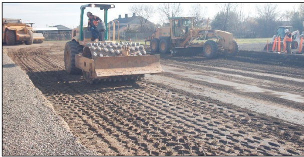
Figure 4.3: Subgrade: Padfoot roller compaction.
