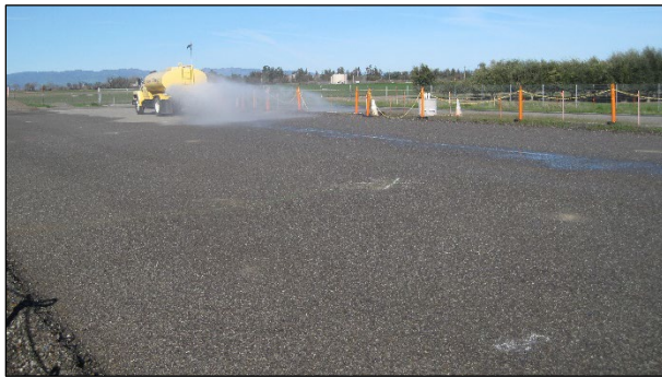
Figure 4.16: Base: Water spray prior to prime coat application.
