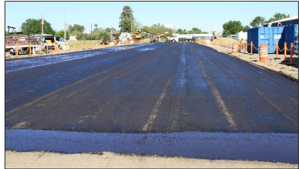
Figure 4.30: CCPR: Completed recycled layer after construction.
