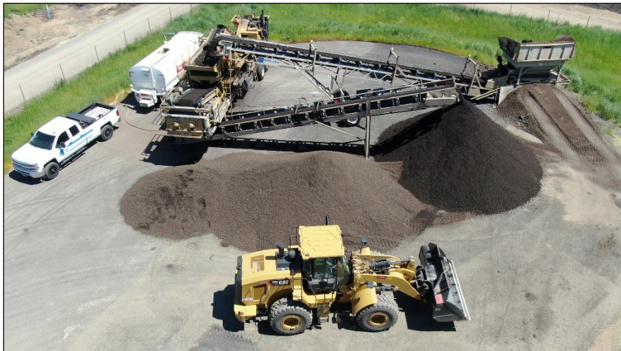
Figure 4.19: CCPR: Screening and crushing setup.
