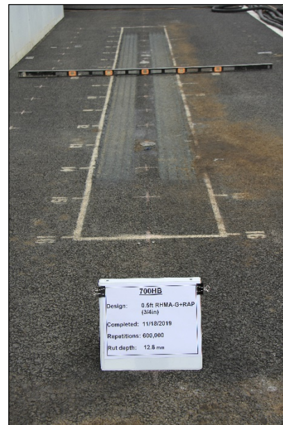
Figure 11.17: 700HB: Test section view from Station 16.
