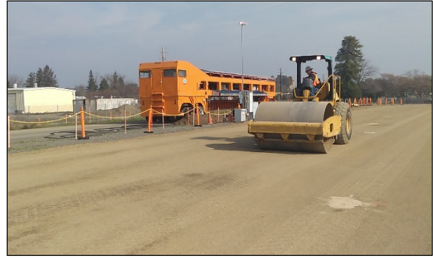
Figure 4.14: Base: Final compaction.
