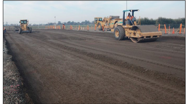
Figure 4.7: Subbase: Spreading and compacting.
