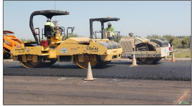
Figure 4.37: RHMA-G: Breakdown (Cell G, front) and intermediate compaction (Cell J).
