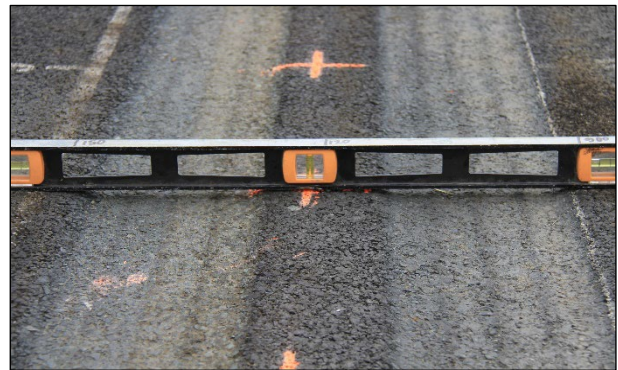
Figure 7.19: 704HB: Close-up view of surface at Station 8.
