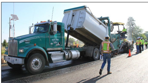
Figure 4.34: RHMA-G: Dumping mix into the paver (Cell J).
