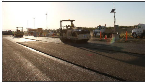
Figure 4.38: RHMA-G: Final compaction (Cells H and I).
