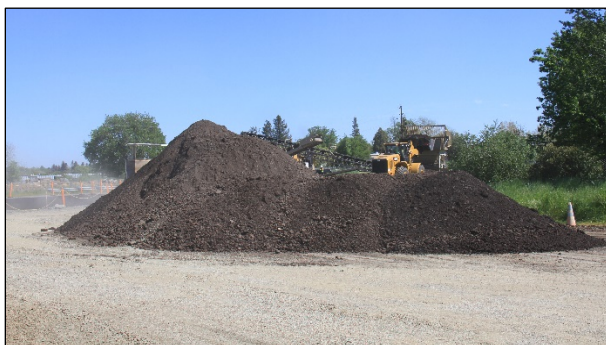
Figure 4.20: CCPR: RAP millings stockpile.
