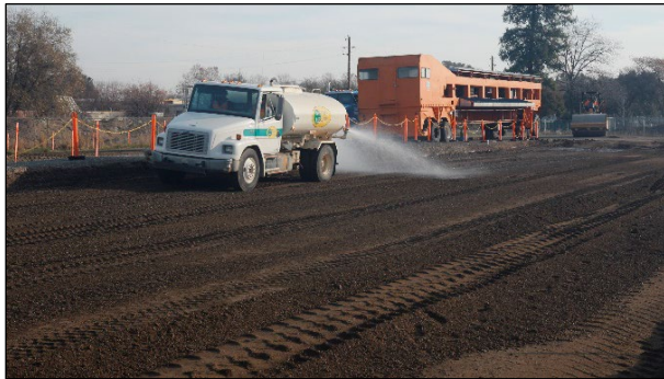
Figure 4.8: Subbase: Water spraying.
