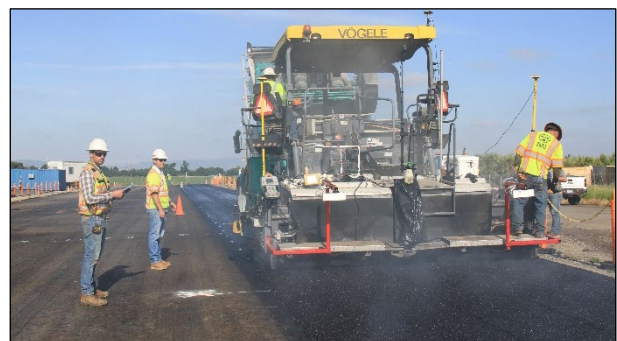
Figure 4.35: RHMA-G: Paving first lift of RHMA-G (Cell J).
