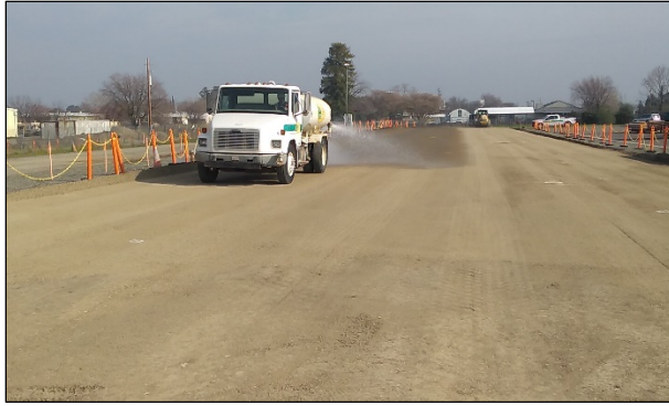
Figure 4.13: Base: Water spraying.
