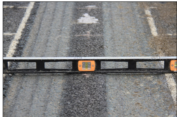
Figure 11.19: 700HB: Close-up view of test section surface at Station 8.
