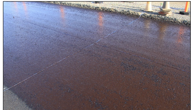
Figure 4.32: RHMA-G: Close-up view of tack coat application.
