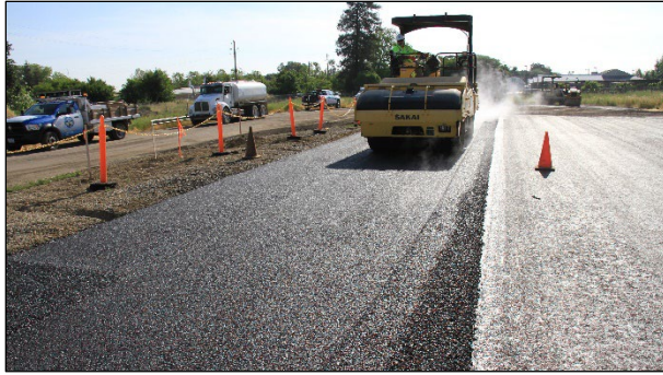
Figure 4.36: RHMA-G: Breakdown compaction (Cell J).
