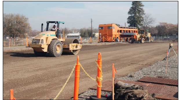
Figure 4.9: Subbase: Final shaping and compaction.
