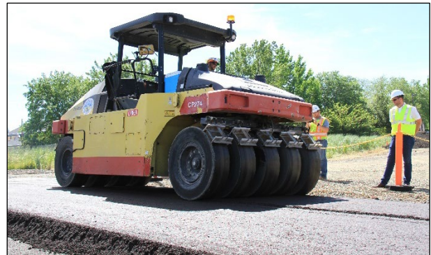
Figure 4.26: CCPR: Intermediate compaction with pneumatic tired roller.
