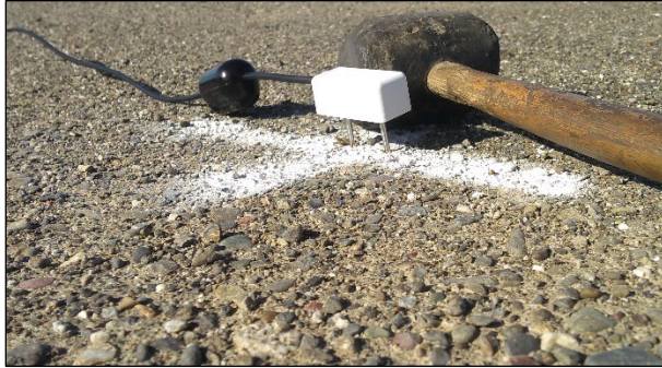
Figure 5.5: Moisture sensor installation on top of subbase.
