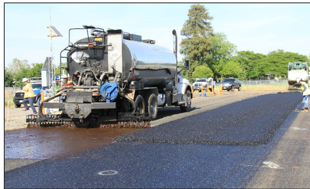
Figure 4.33: RHMA-G: Tack coat application between lifts of RHMA-G (Cell J).
