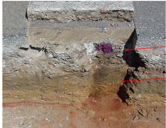
Figure 3.14: Phenolphthalein reaction on base.
