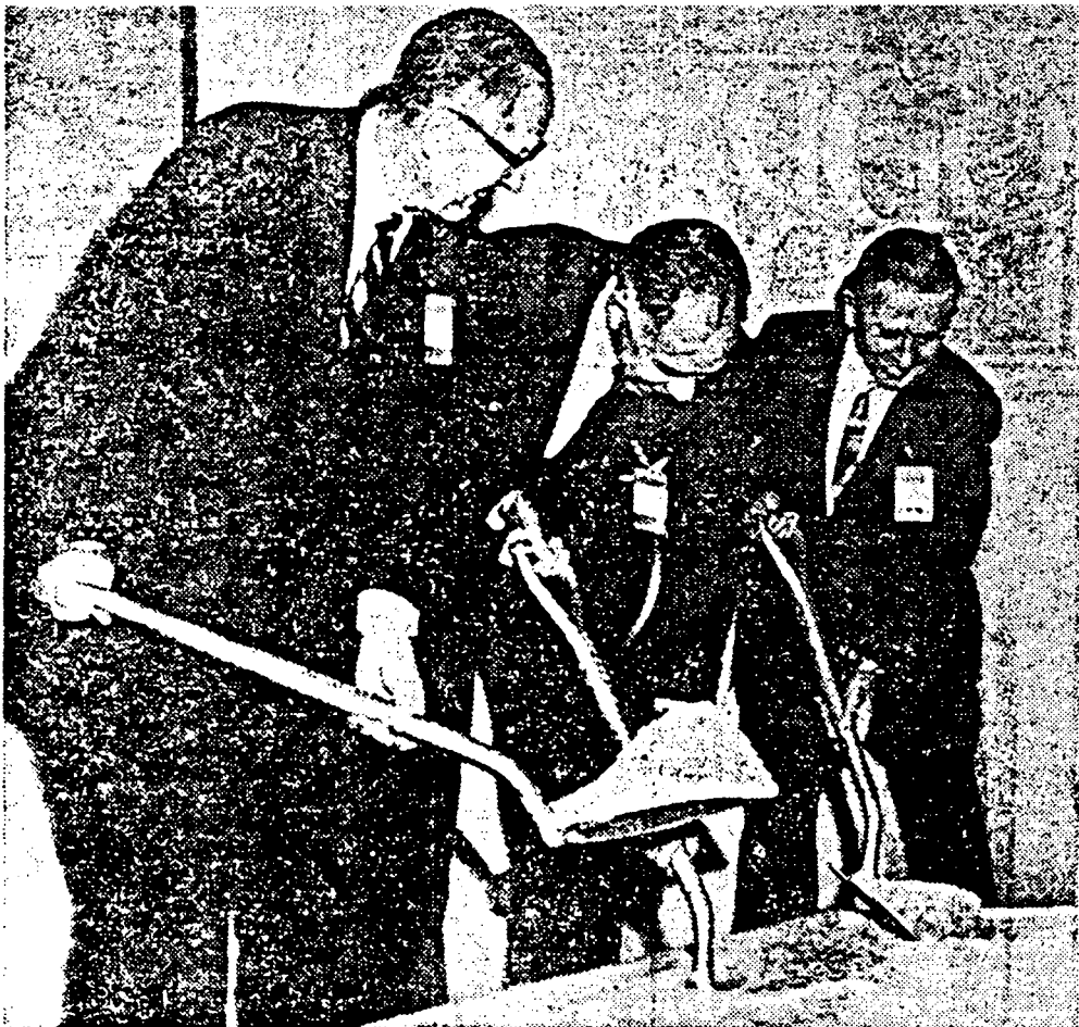
Snow moved the groundbreaking for the Los Alamos Meson Physics Facility indoors but gold-plated shovels wielded by U.S. Sen. Clinton P. Anderson,
