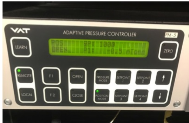
Figure A.14: VAT controller which sets the position of the gate valve that sits in front of the turbo pump (visible through the viewport). During normal operation, the gate is fully in the open position. Closing it will increase the chamber pressure.
