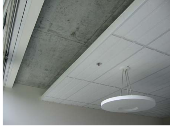
Figure 6. Acoustical Tile Ceiling Cloud
