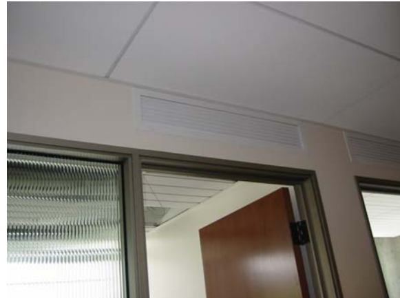
Figure 8. Offset Return Air at Open Plan
