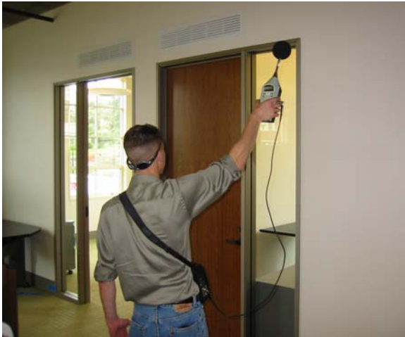
Figure 16. Sound Leak Assessment
