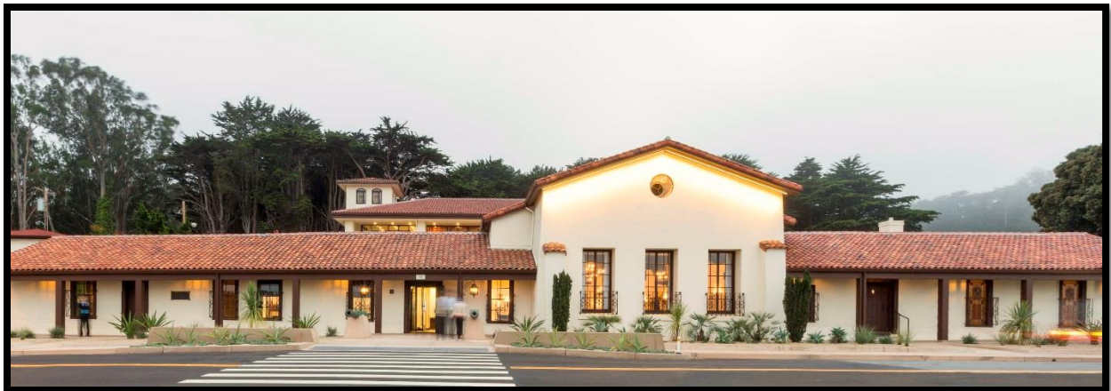
Figure 23: Photograph of the Officers' Club today. The two low wings flanking the taller main hall are what remain from the colonial adobe. The rest of the structure is composed of various additions from the main hall at the central façade constructed in the 1880s to the large two story addition and tower (center background constructed in the 1970s. )
