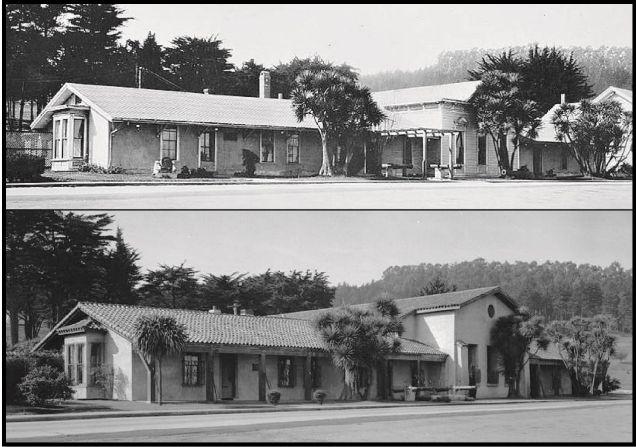
Figure 27: Photographs of the Officers' Club before (above) and after (below) restoration efforts in 1934 (courtesy of PARC).
