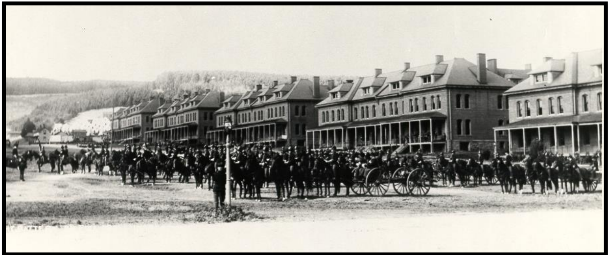
Figure 5: The Montgomery Street barracks for enlisted men pictured shortly after their construction with soldiers on the drilling field in the foreground (courtesy of PARC).
