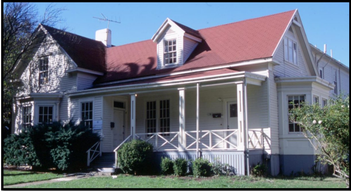
Figure 1: One of the empty homes along Officers' Row prior to rehabilitation to be repurposed as offices (image courtesy of the Presidio Trust).
