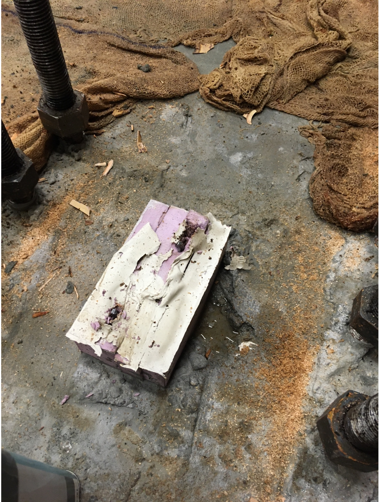
Figure F- 50. Removing plywood anchor molds
