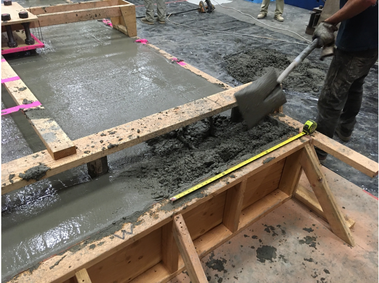
Figure F- 44. Casting concrete
