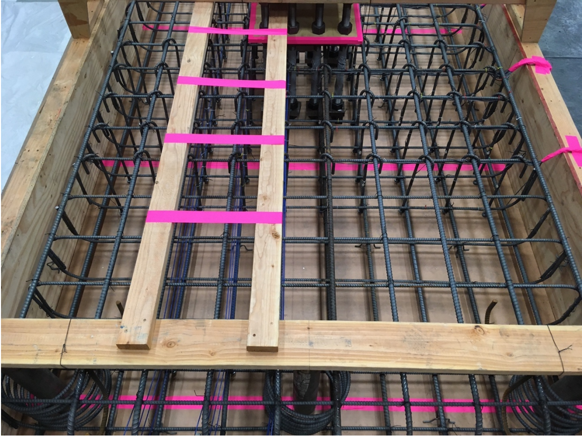
Figure F- 28. Form before casting concrete
