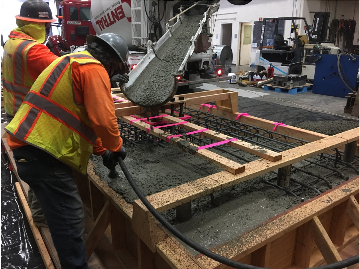
Figure F- 33. Casting concrete
