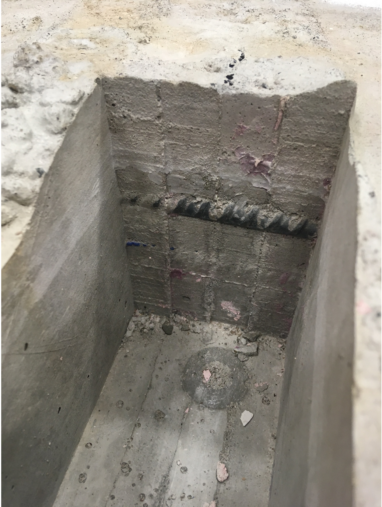
Figure F- 60. Hole left by foam mold for shear lug
