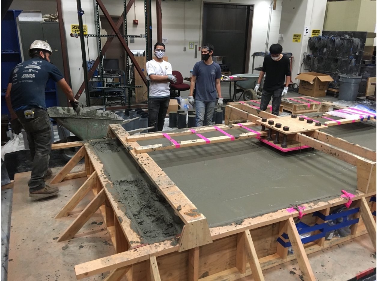
Figure F- 43. Casting concrete
