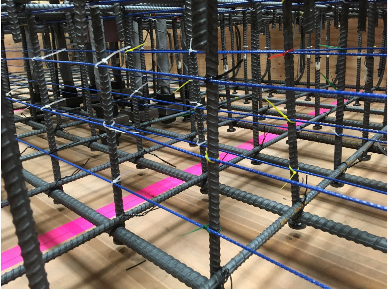
Figure F- 17. Placement of fiber optics cables
