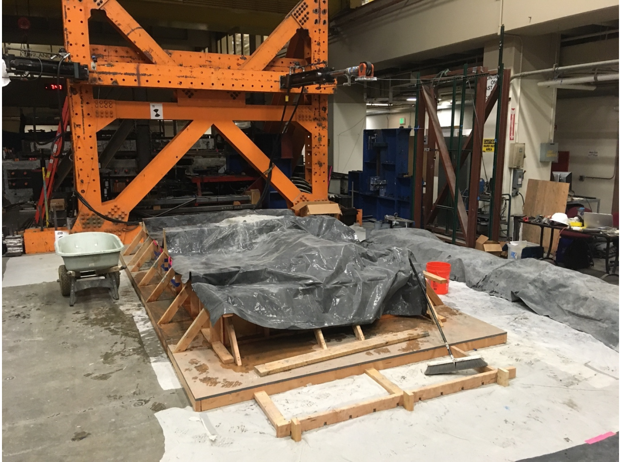
Figure F- 49. Curing specimen and cylinders with burlap and plastic
