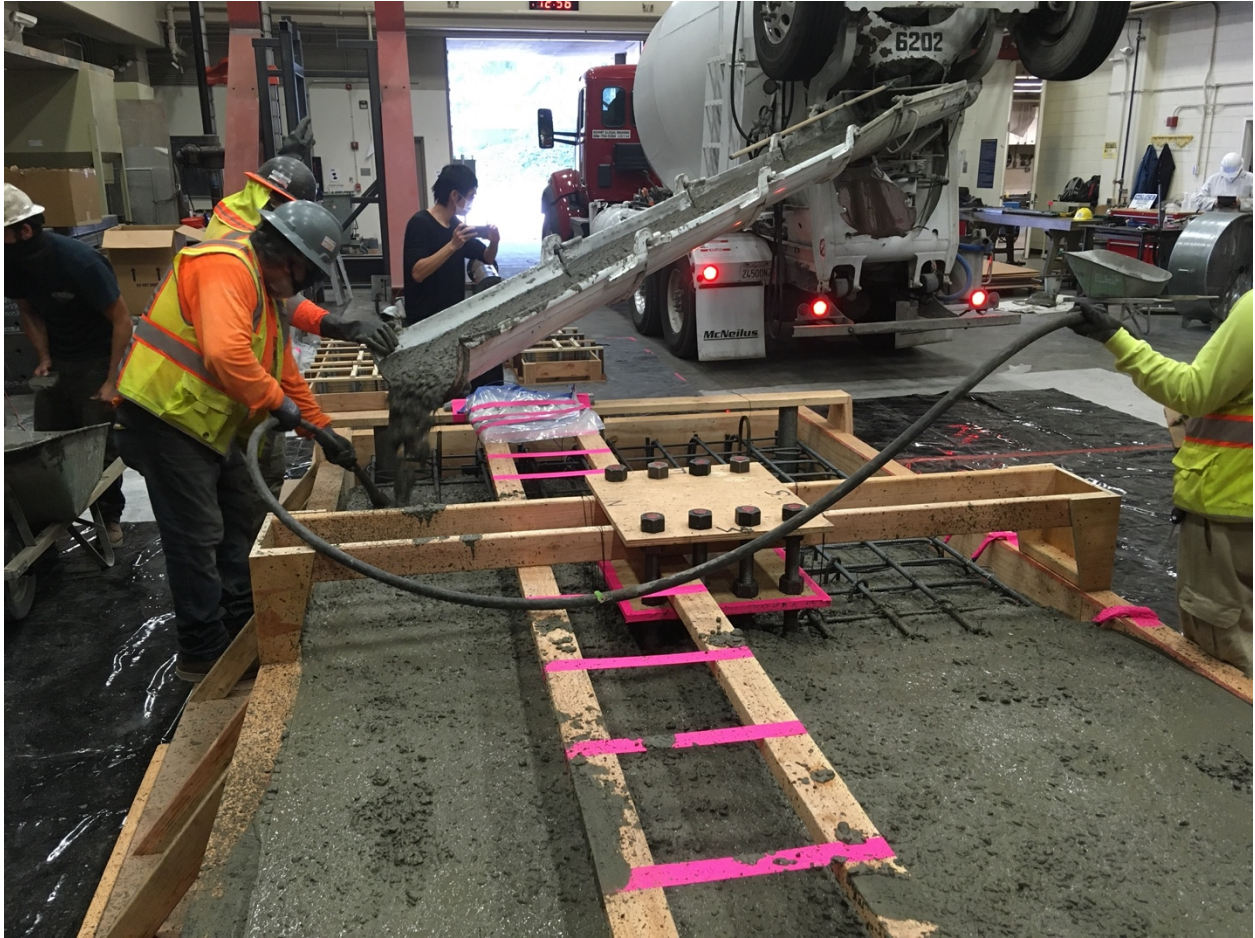
Figure F- 35. Casting concrete
