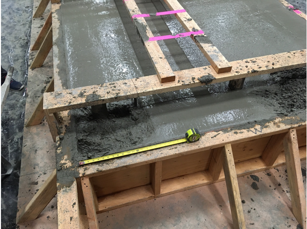
Figure F- 45. Casting concrete
