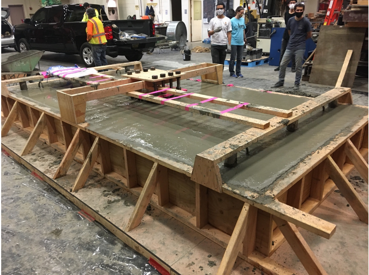
Figure F- 47. Casting concrete
