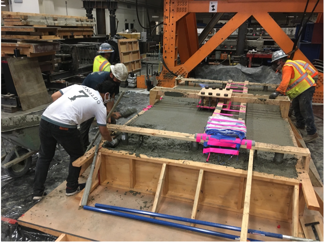
Figure F- 38. Casting concrete
