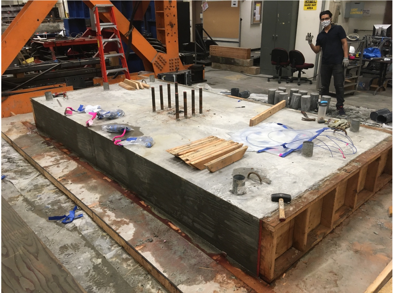
Figure F- 52. Removing formwork
