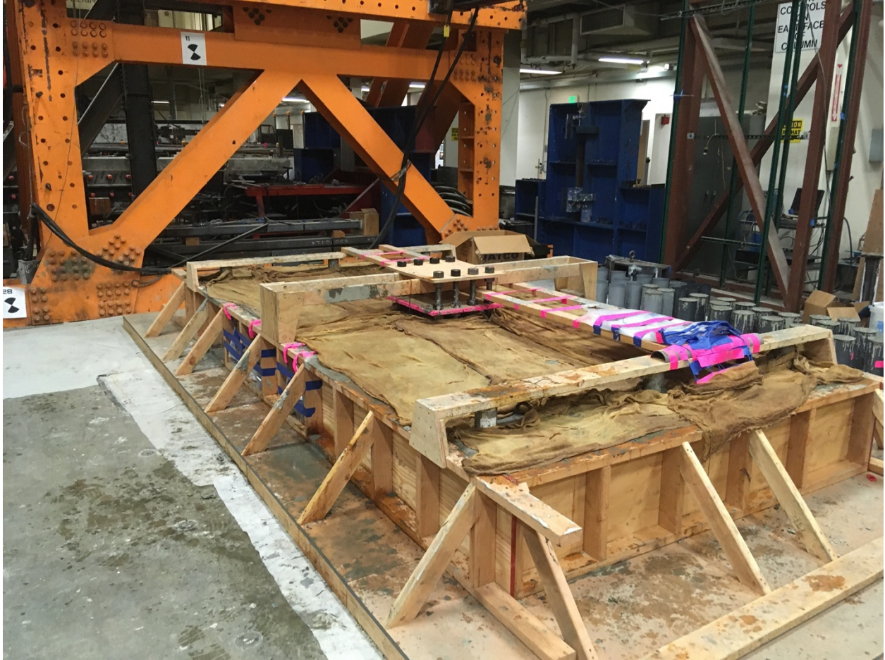
Figure F- 48. Curing specimen with burlap
