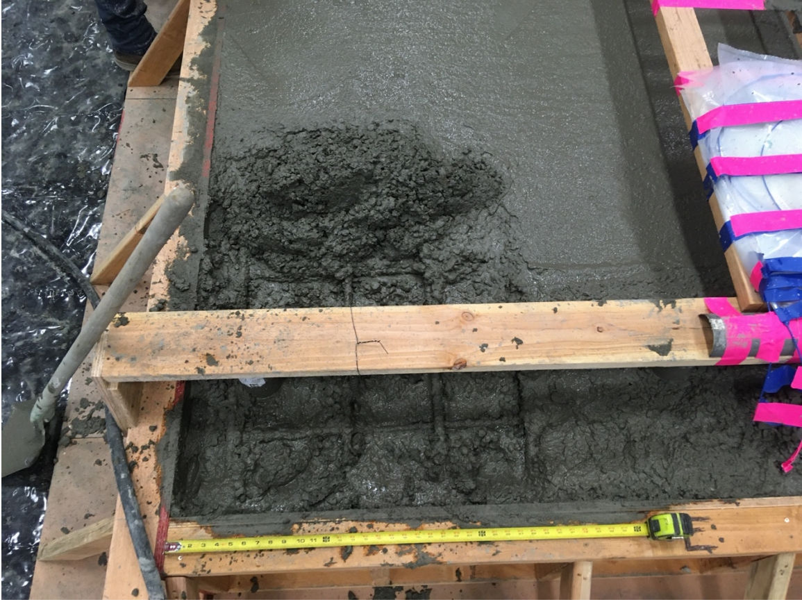
Figure F- 41. Casting concrete
