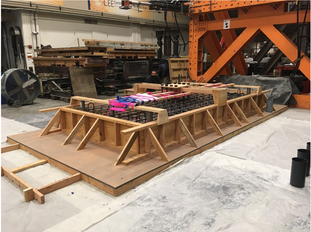
Figure F- 25. Form before casting concrete
