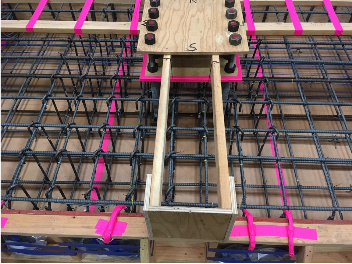
Figure F- 29. Form before casting concrete
