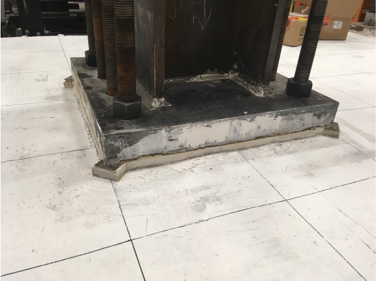
Figure F- 62. Column hydrostoned to specimen
