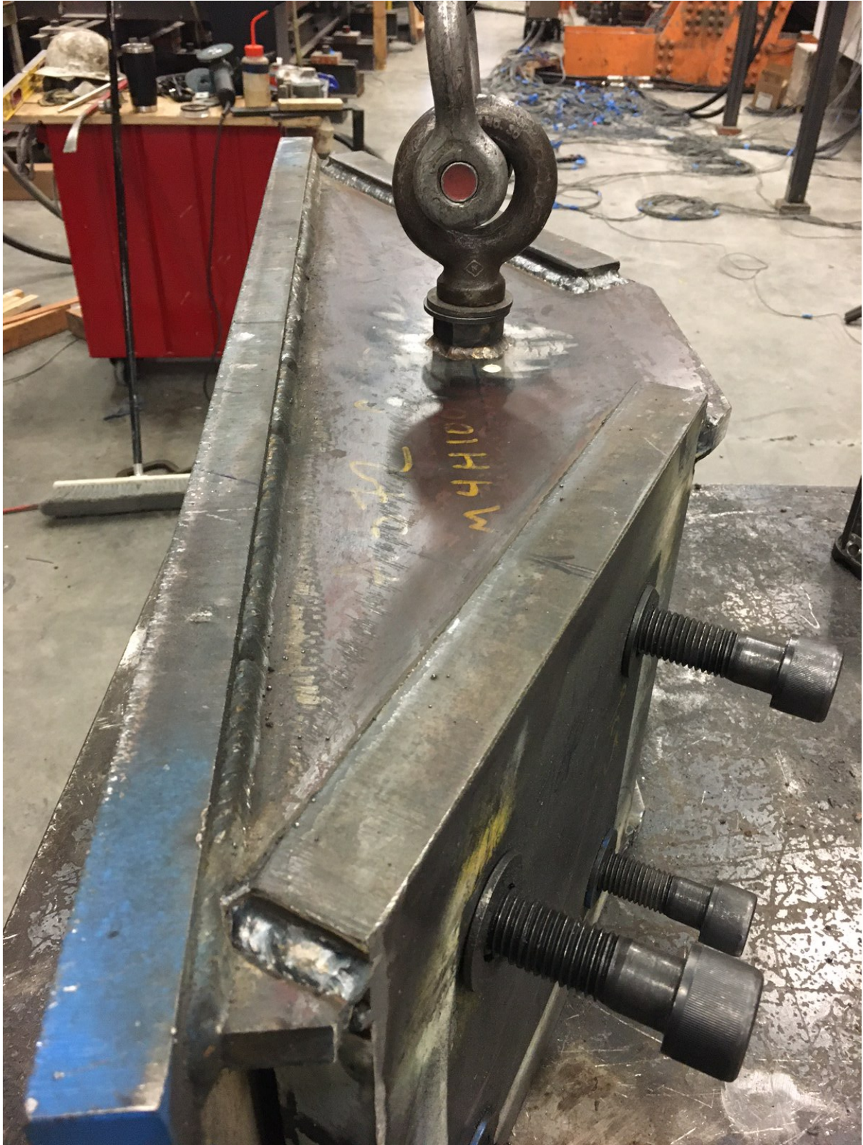
Figure F- 68. Modification to column-actuator attachment
