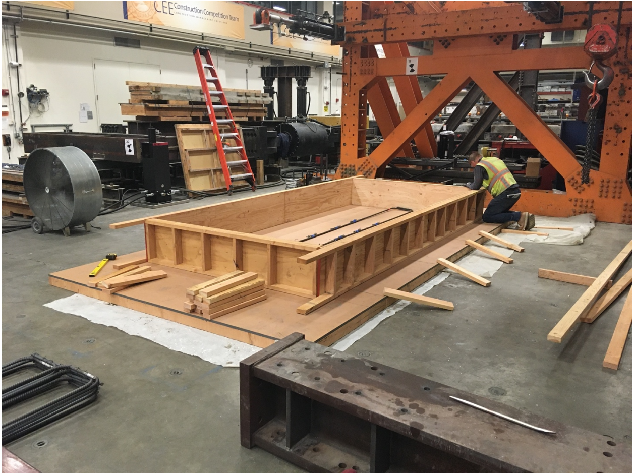
Figure F- 8. Form building
