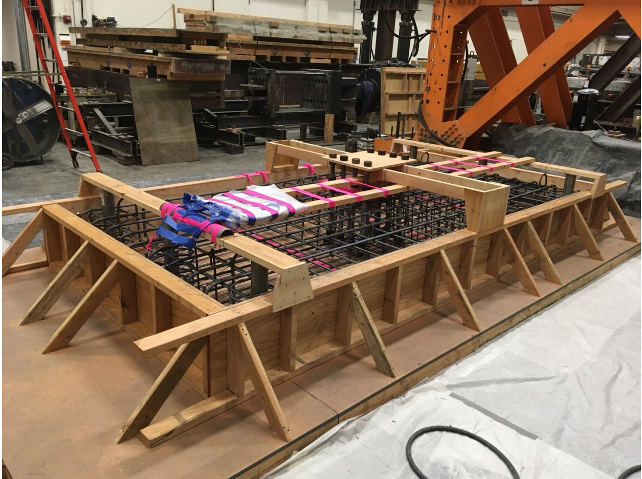
Figure F- 18. Form before casting concrete
