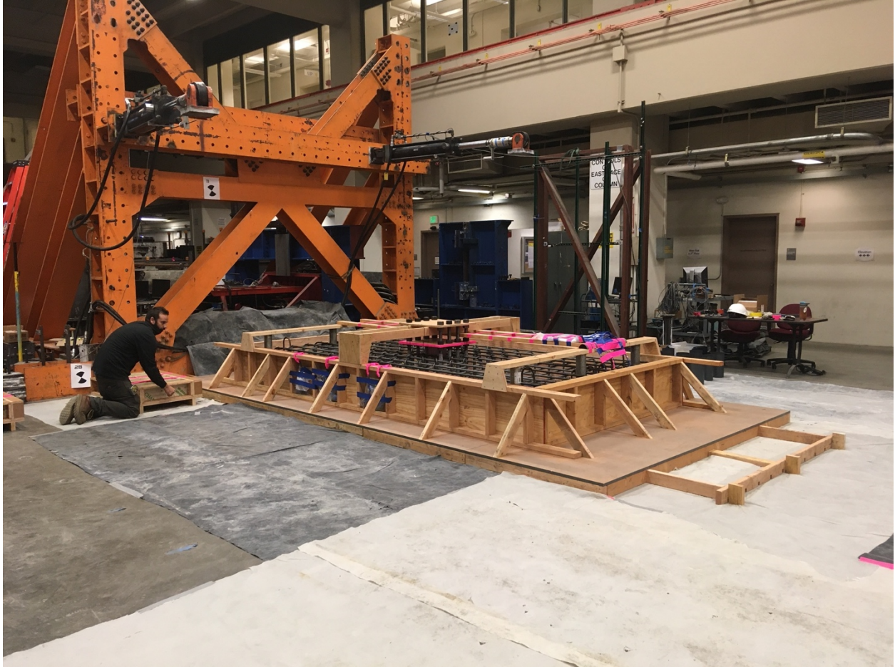
Figure F- 26. Form before casting concrete
