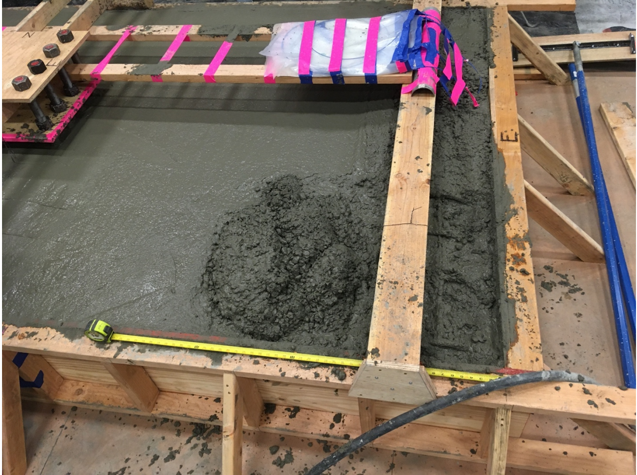
Figure F- 42. Casting concrete
