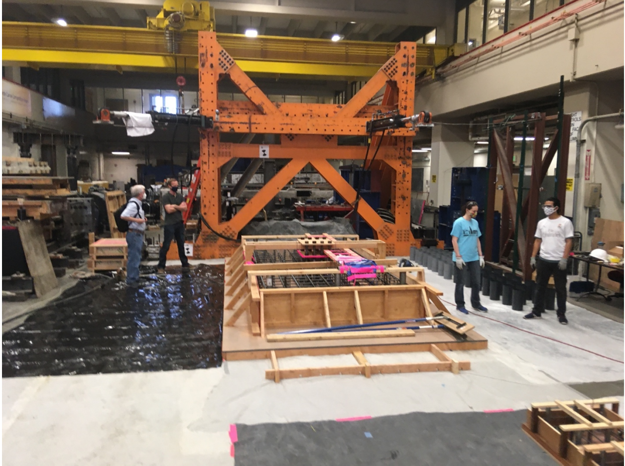
Figure F- 31. Form before casting concrete
