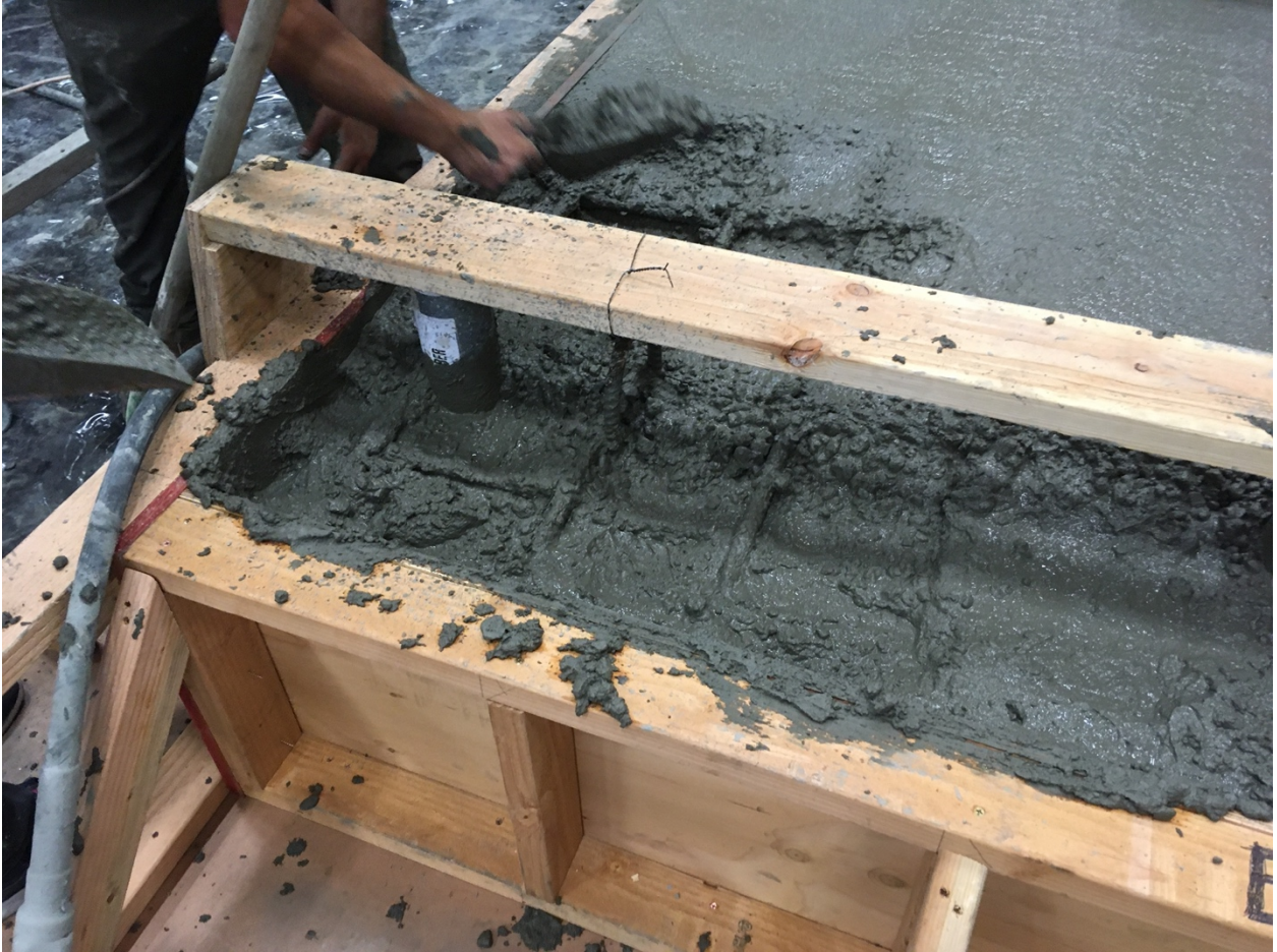
Figure F- 40. Casting concrete
