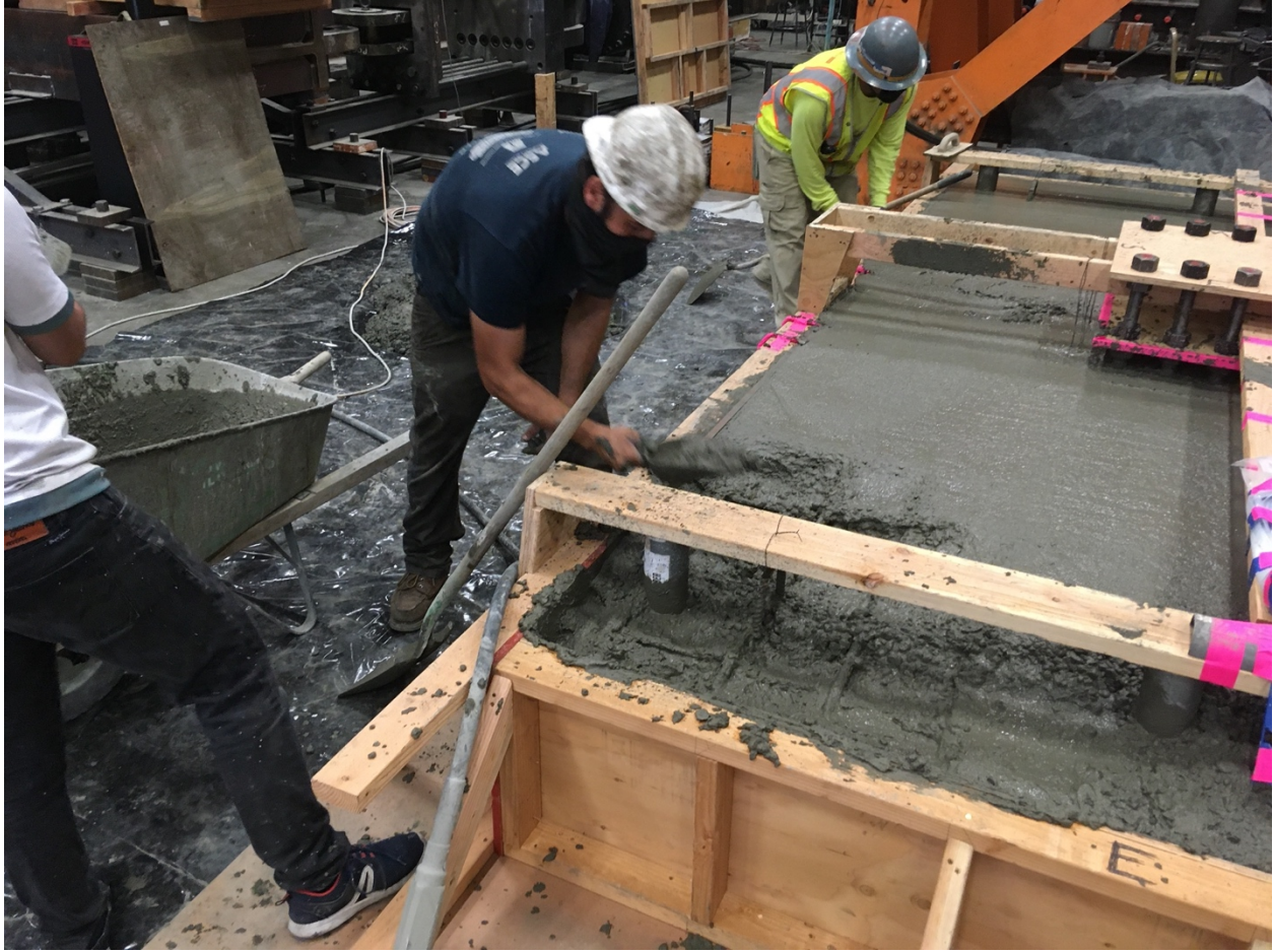
Figure F- 39. Casting concrete
