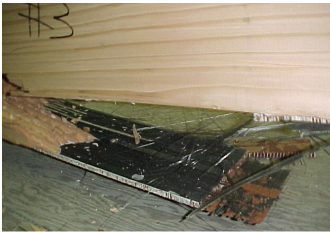
Fig. 18. Cohesive failure of beams retrofitted with sandwich composite laminates indicating proper interfacial bond between wood and composites.
