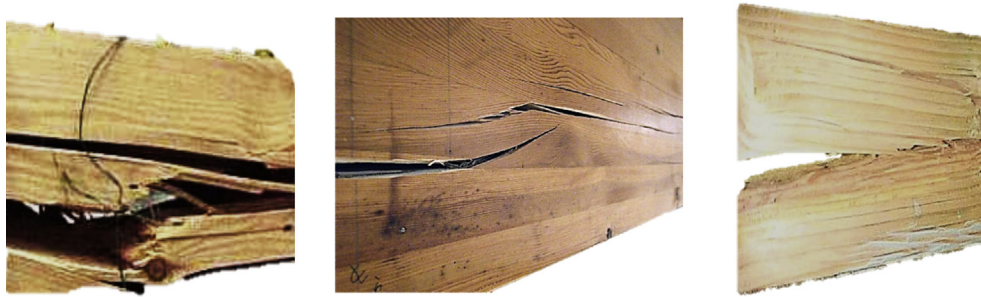
Fig. 2. Interlaminar shear failure of wood members subjected to flexure.
