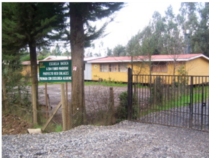
Figure 2.10: A classroom building on site at one of the public primary schools in Makewe
