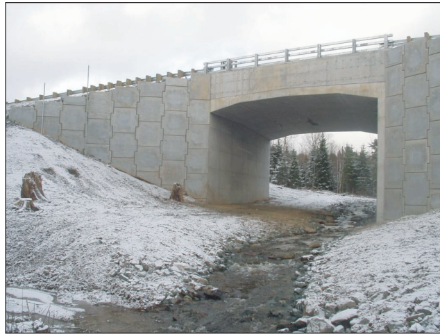
Figure 2. Doyon Creek concrete box culvert before tree and shrub planting.
