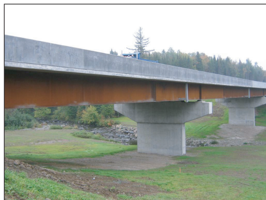
Figure 3. Calway River open-span Bridge before tree and shrub planting.
