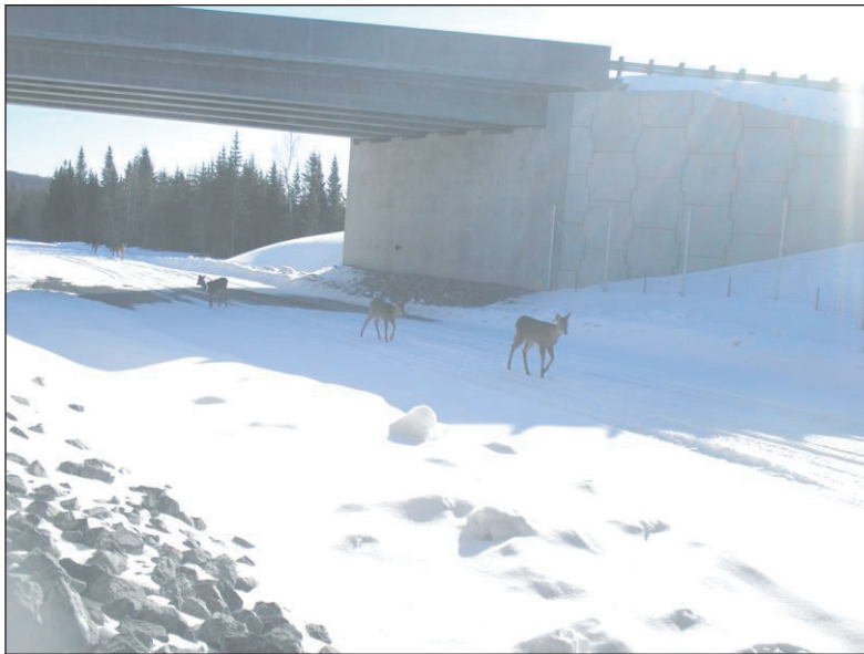
Figure 10. Six deer passing under the Carrière Road bridges, a secondary deer crossing underpass on 10 April 2007.
