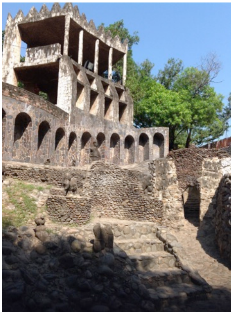
Figure 35: Fortress structure in Phase I [photograph by the author, 2014]
