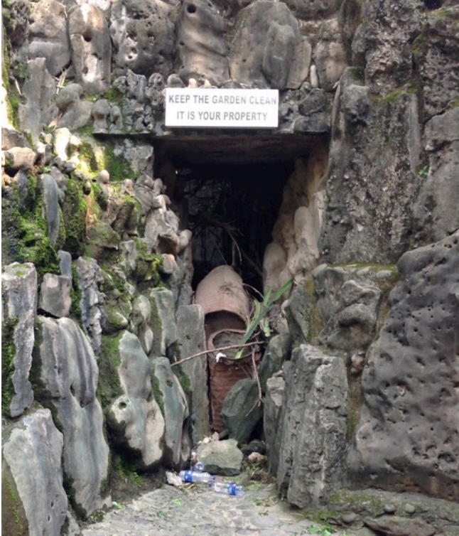
Figure 10: Path blocked by rocks and bitumen drums [photograph by the author, 2014]
