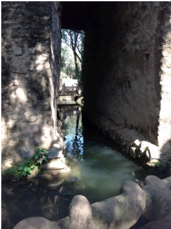
Figure 31: View from pathway into Phase III [photograph by the author, 2014]
