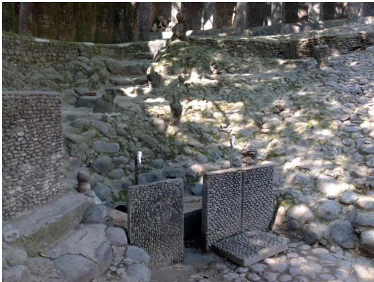
Figure 33: Stone basin, steps, and partition walls [photograph by the author, 2014]
