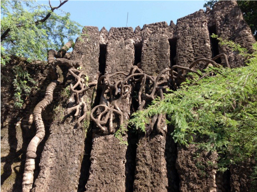
Figure 95: Concrete "roots" [photograph by the author, 2014]
