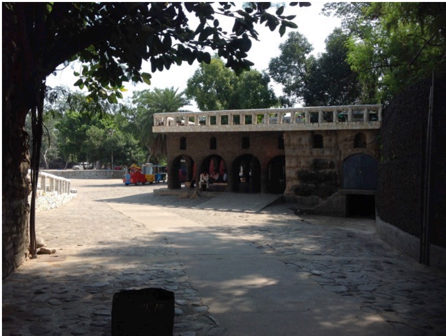
Figure 57: View of Phase-III building from walkway [photograph by the author, 2014]
