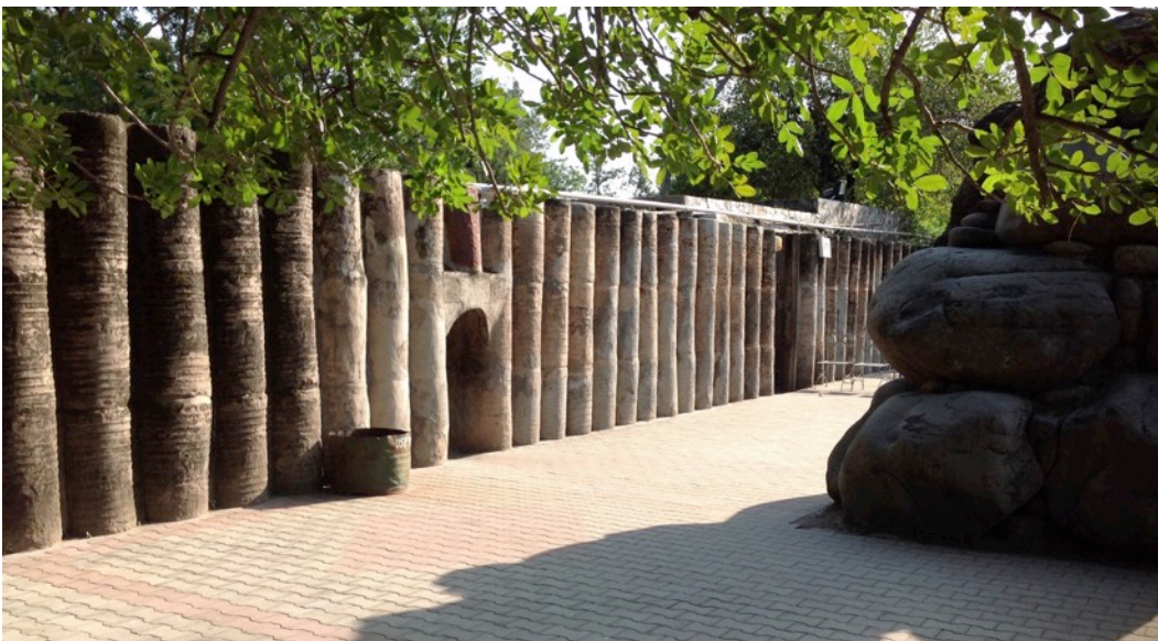
Figure 2: Stacked bitumen drums as site border wall [photograph by the author, 2014]
