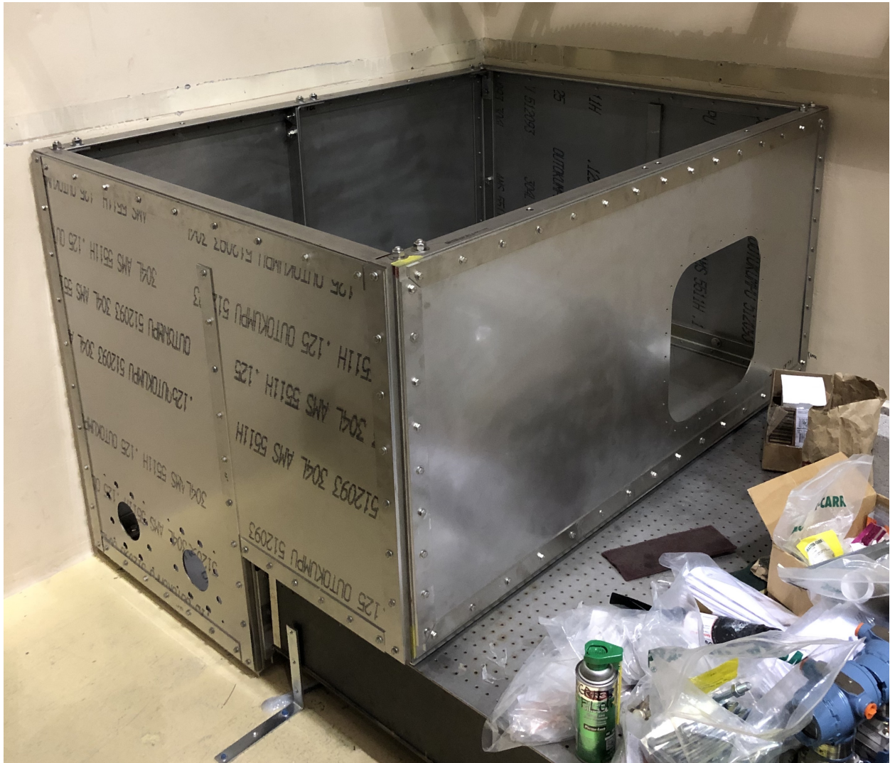
Figure 3.2: The stainless steel discharge tank assembled in place, prior to being sealed. Water enters from the test section through the hole on the right side of the figure. The two holes at the bottom left are outlets that lead to the suction side of the pumps.
