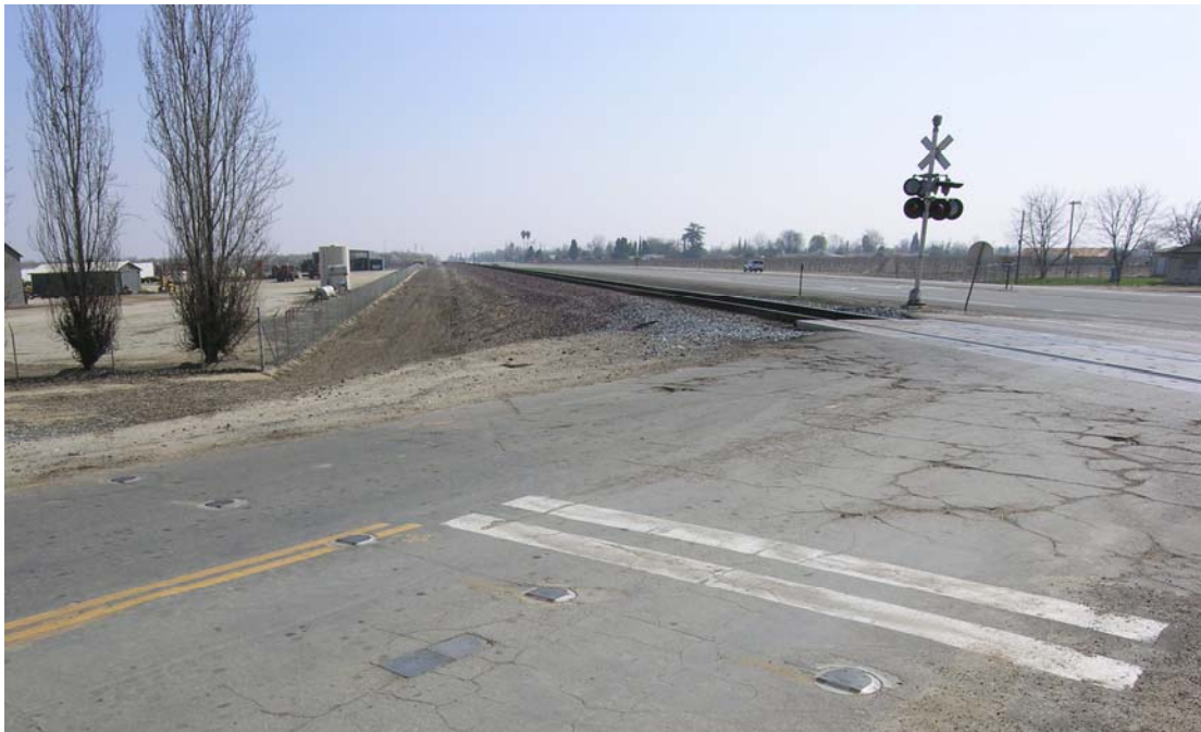
Figure 9: The same five embedded lights as seen from above and looking more easterly.
