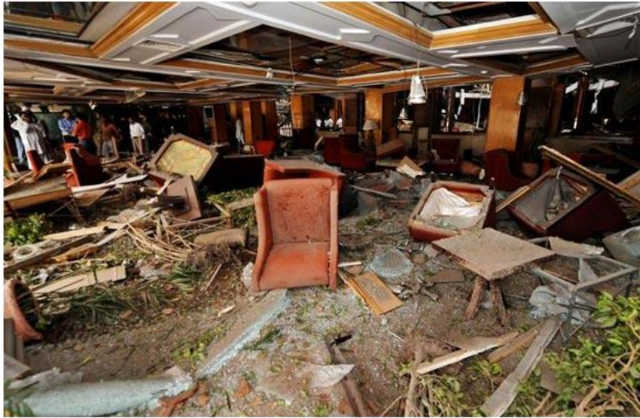
Workers inspect the inside of the shattered hotel.
