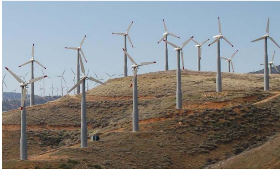
Figure 2.3: Field installation at Oak Creek Energy Systems in Tehachapi, California, USA
