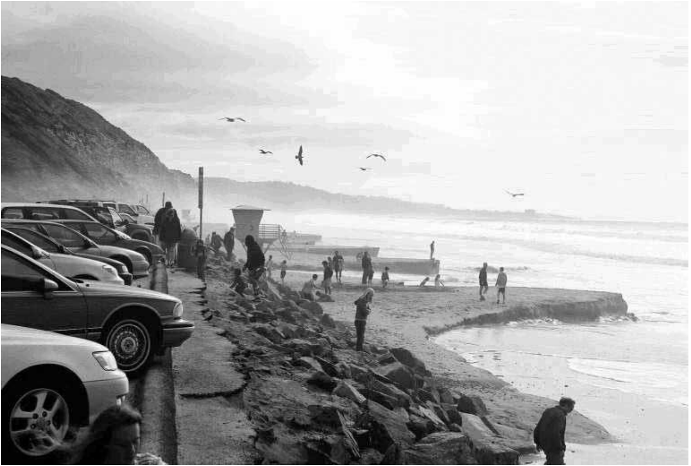
Figure 15. Beach fill erosion as a series of embayments
