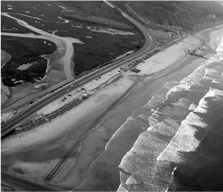
Figure 2. View of the beach fill site showing the Torrey Pines cliffs to the south and the lagoon mouth to the north.
