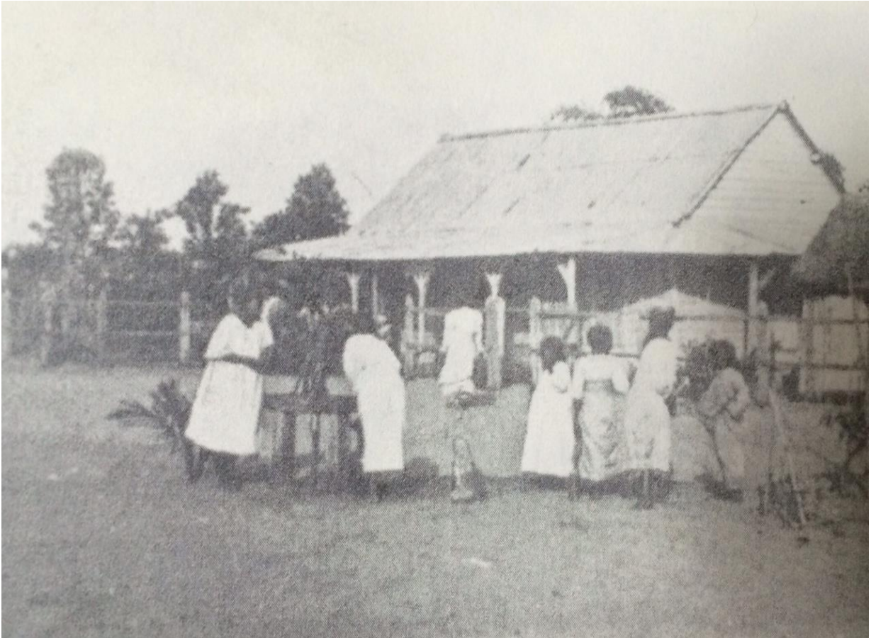
Figure 2.1. Police station in the “indigenous village” of Toamasina, an example of infrastructure built by the colonizers to regulate the population, c. 1900.
