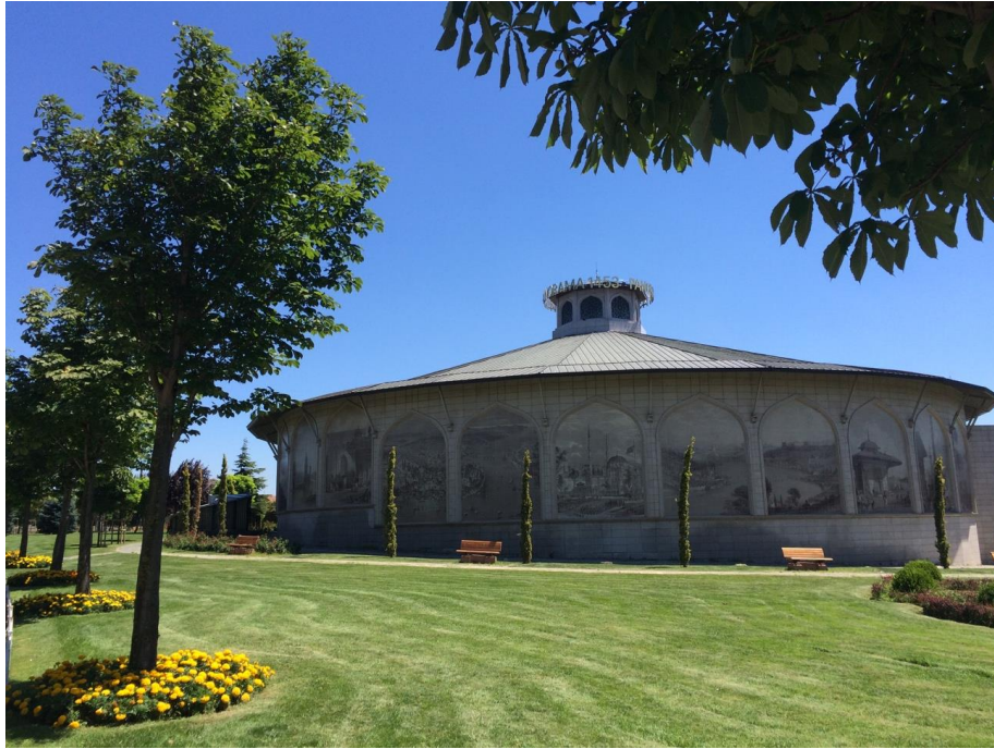
Figure 8.2. External view of the Panorama 1453 Historical Museum building . July 2016. Istanbul. Photo: Ayda Melika.
