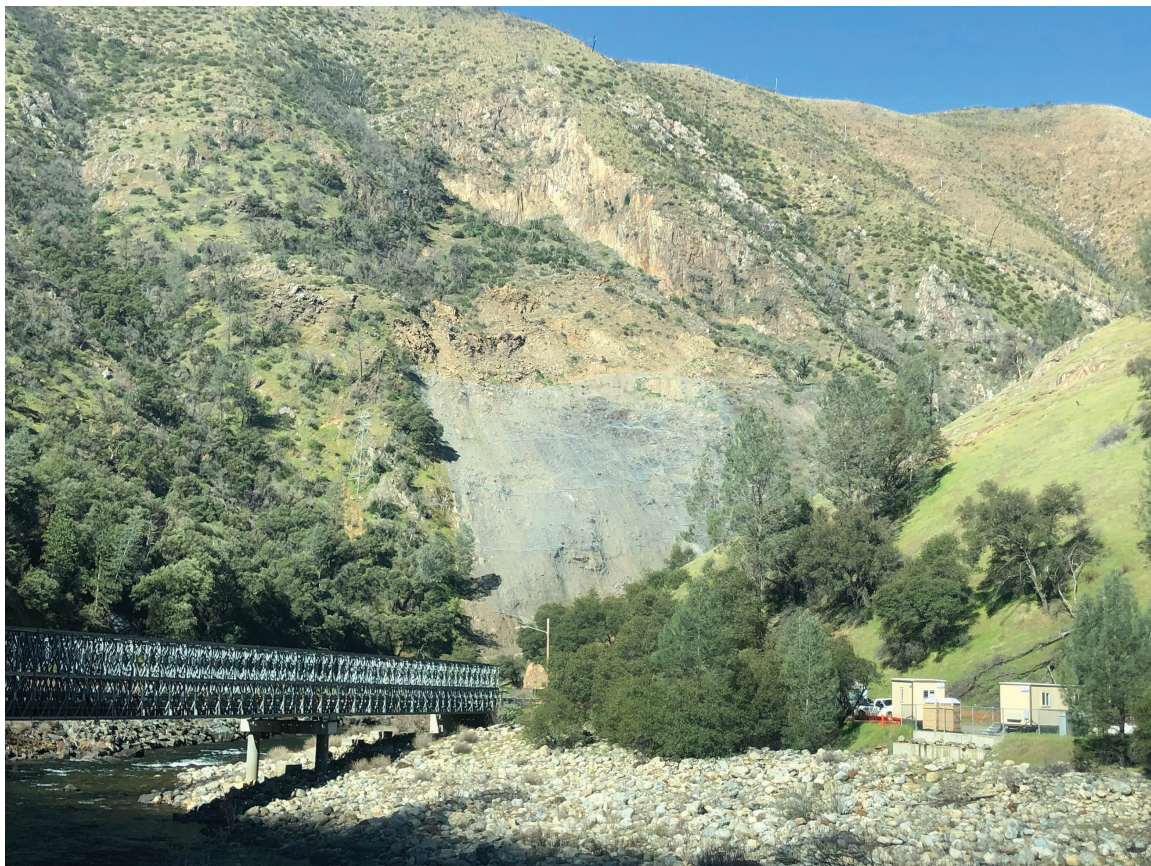
FIGURE 7. The Ferguson slide and temporary bridge for Highway 140 crossing the Merced River. JEFFREY JENKINS
