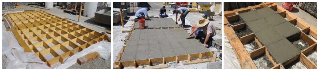
(a) Plywood formworks (b) Normal weight concrete (c) Higher strength concrete
