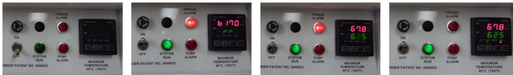
Figure A.2: From left to right, showing the state of chiller before and after Power ON.
