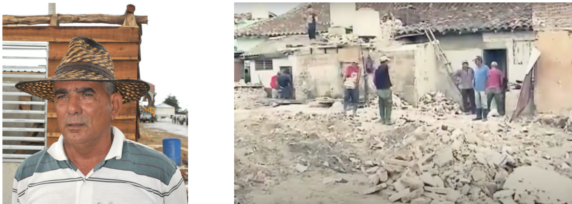
Figure 4. 10: The work of reconstruction of Emilio Cordoba
