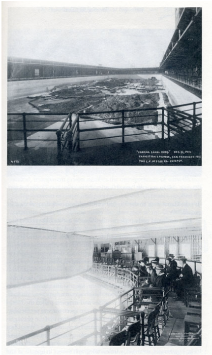
Fig. 16: Top: Model of the Panama Canal at the Panama Canal exhibit Bottom: Spectators gallery at the Panama Canal exhibit
