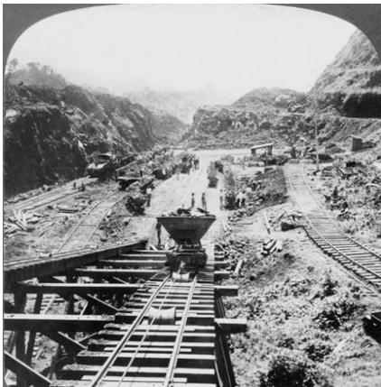
Fig. 1: Panama Canal under construction (1907)
