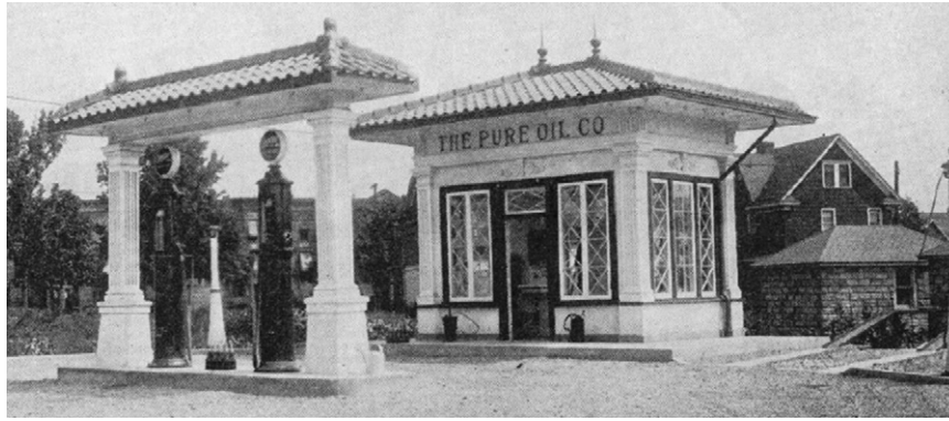
Fig. 9. A Pure Oil Company steel prefabricated station (National Petroleum News, 3 November 1926, p. 48G-H).
