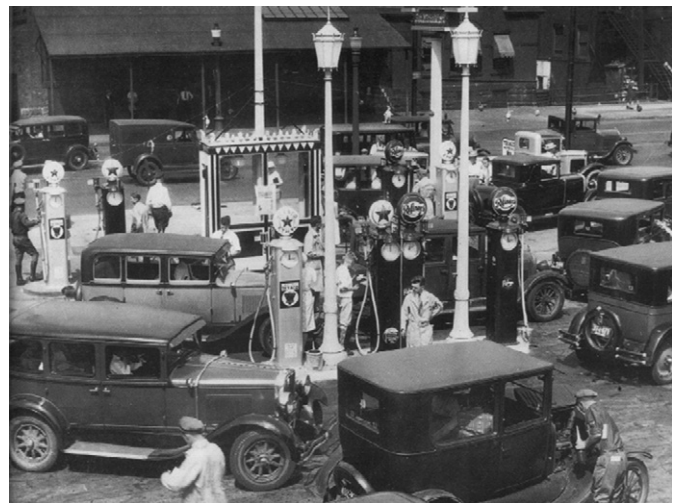
Fig. 7. Curb pumps on a busy street corner (Margolies, 1993, p. 121).
