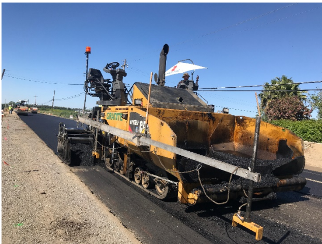
Figure 4.9: Asphalt placement and compaction.
