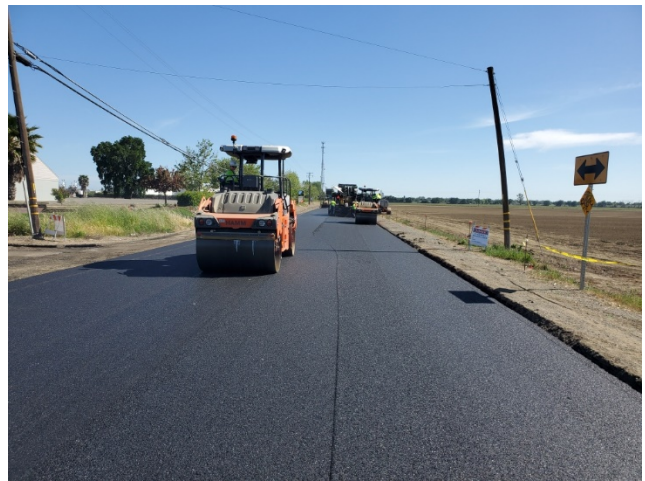
Figure 4.9: Asphalt placement and compaction.
