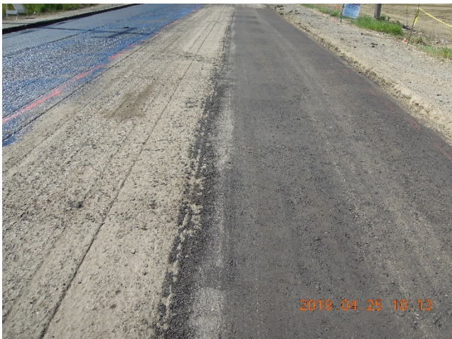
Figure 4.5: Asphalt patching on areas with insufficient or missing asphalt base.
