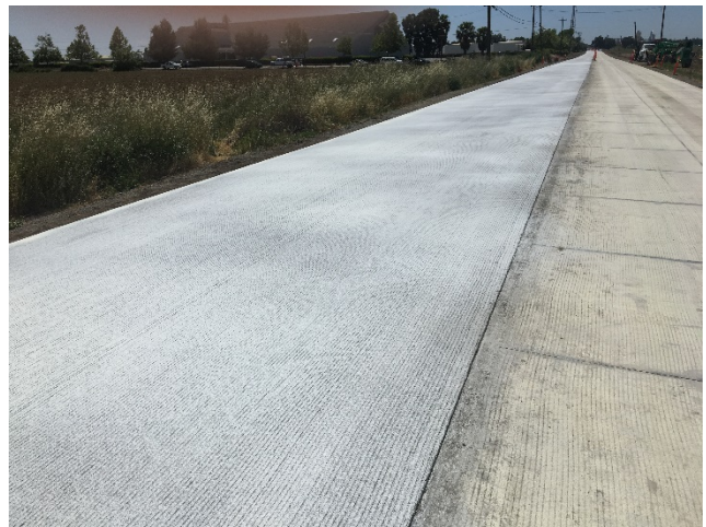
Appearance of the final surface
