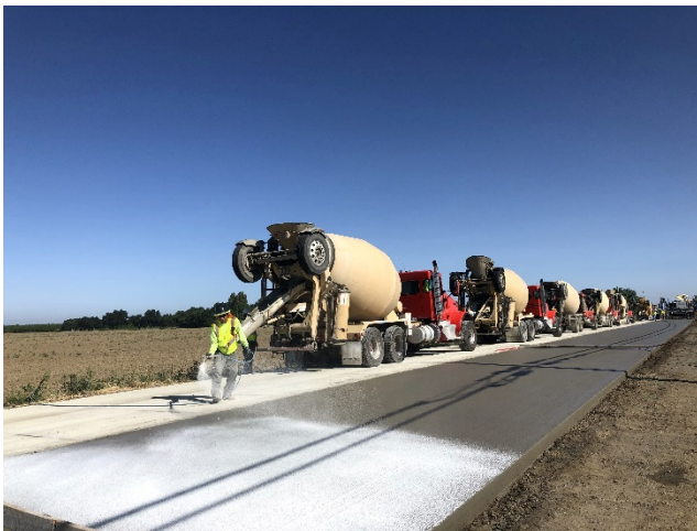
Manual spraying of curing compound
