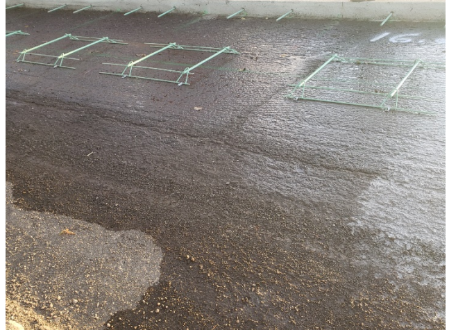
Figure 4.12: Dirt on the asphalt surface before concrete paving.
