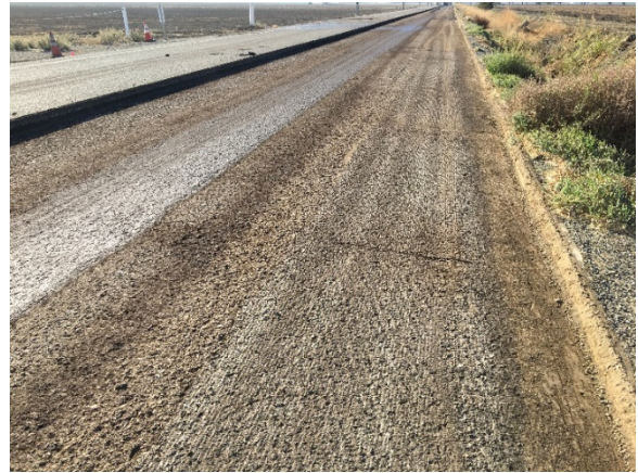
Segment B: Asphalt cracking and areas with delamination
