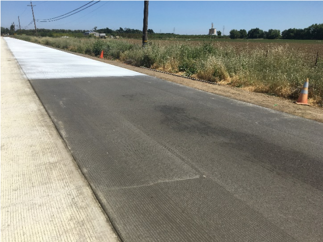
Surface appearance before SRA application
