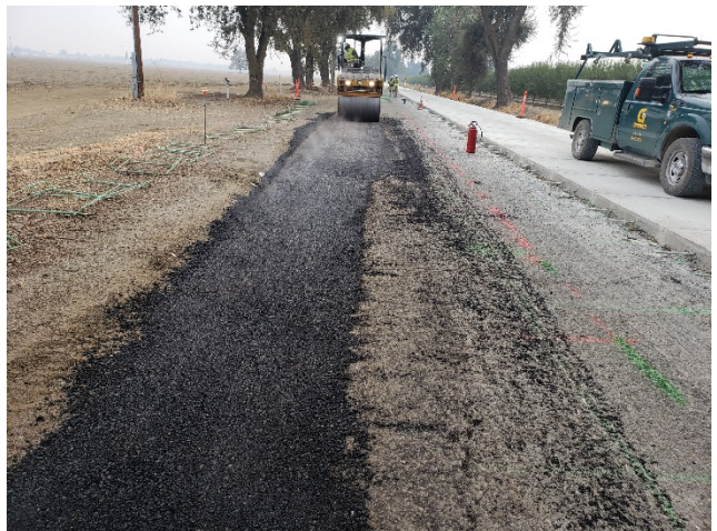
Figure 4.5: Asphalt patching on areas with insufficient or missing asphalt base.
