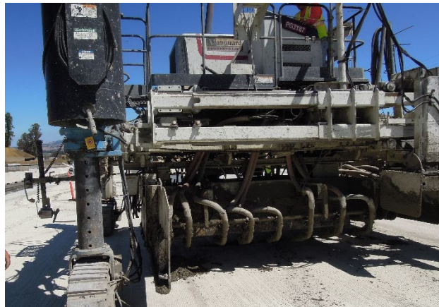
Figure 3.4: Vibrators of the paving machine.
