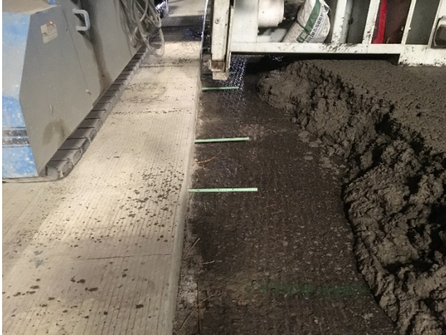
Figure 4.12: Dirt on the asphalt surface before concrete paving.
