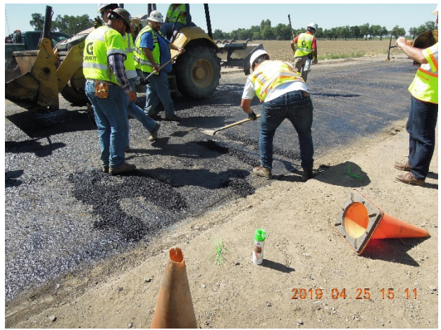
Hot RHMA-G placed over the strain gauges and cables right before the RHMA-G extension
