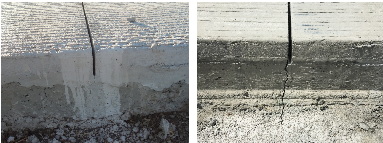
Figure 4.34: Deployed transverse joints.
