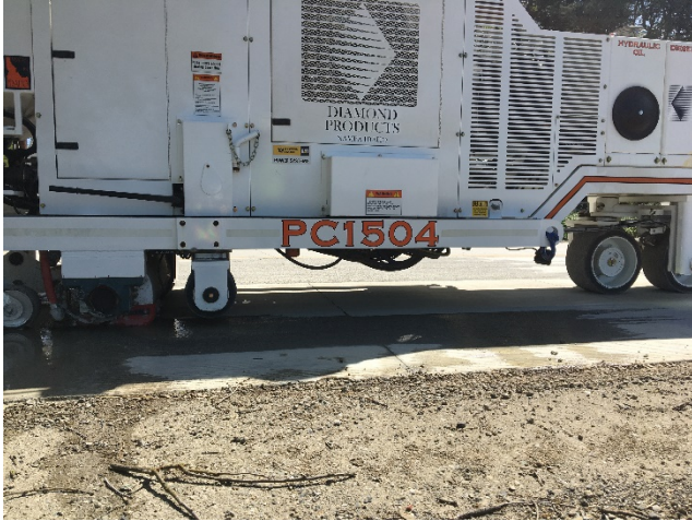
Concrete surface grinding
