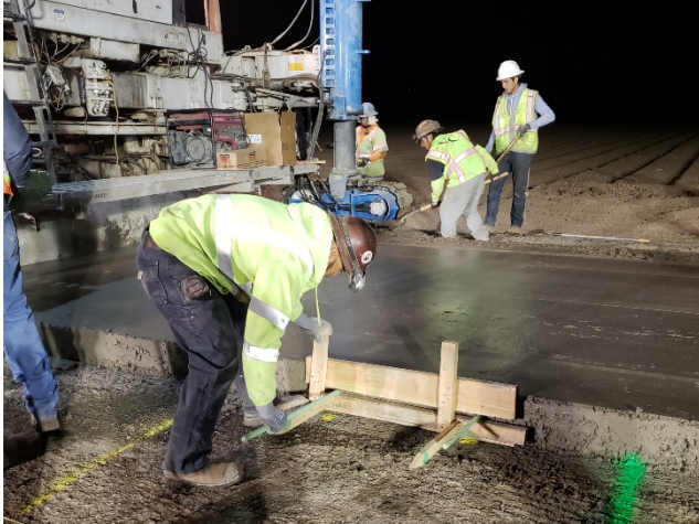
Manual insertion of tie bars in the plastic concrete
