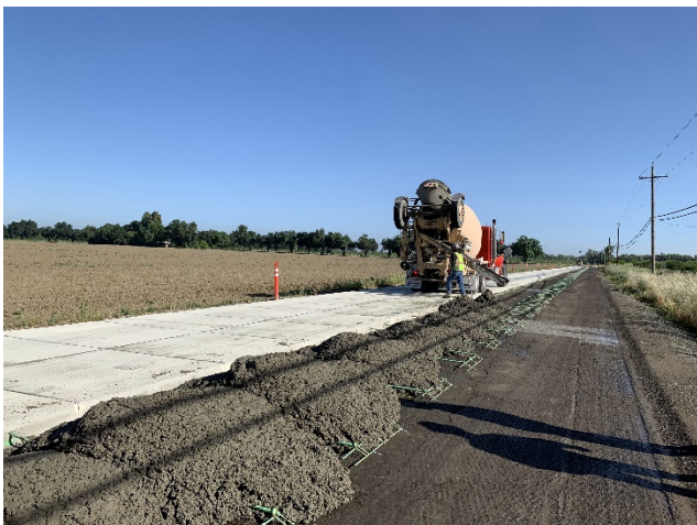
Asphalt surface is adequately wet conditioned: uniformly moist but free of standing or flowing water
