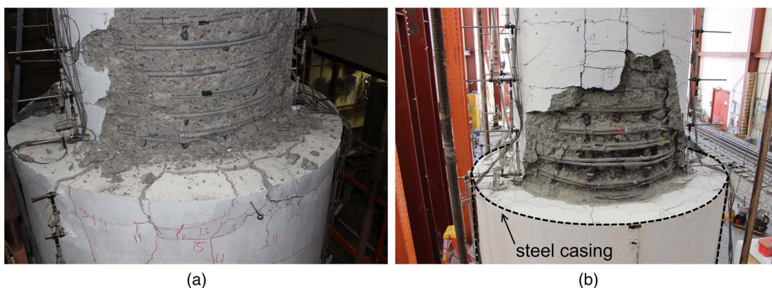
Fig. 2. Damage in the column-pile specimens at the end of testing (reprinted from Murcia-Delso et al. 2016, © ASCE): (a) Specimen 2; (b) Specimen 3
